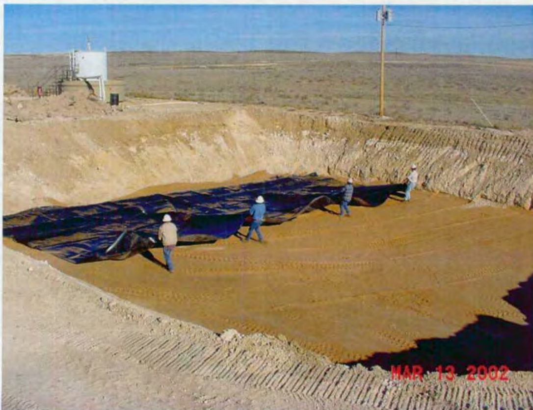
Bottom Photo: Pit 2 excavation, laying out liner.
