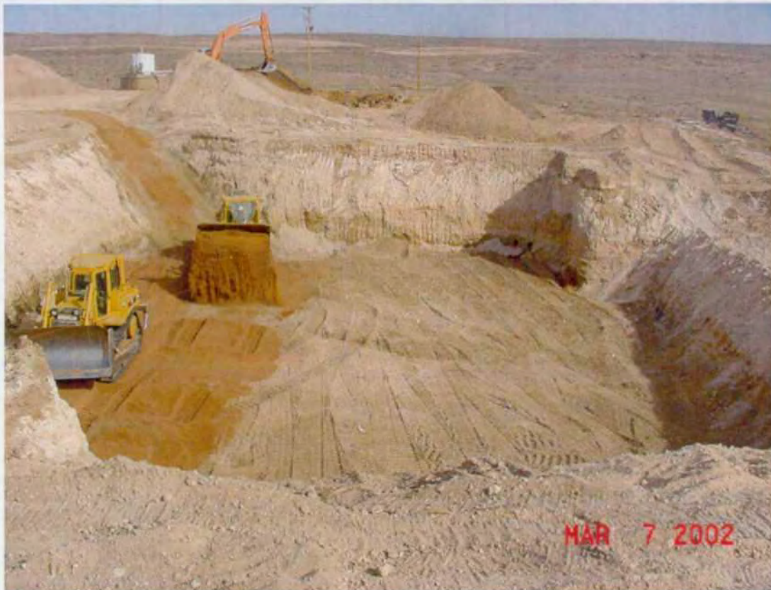
Top Photo: Pit 1 excavation, preparing bottom for liner.
