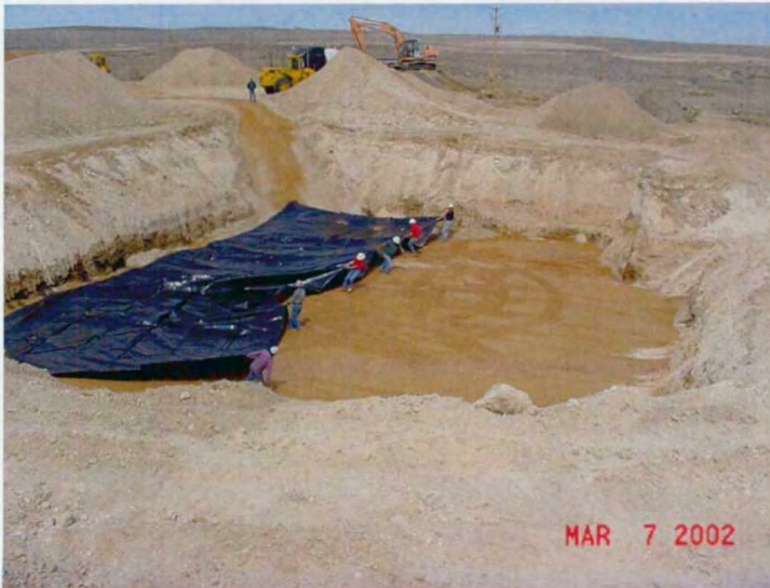
Bottom Photo: Pit 1 excavation, laying out liner.
