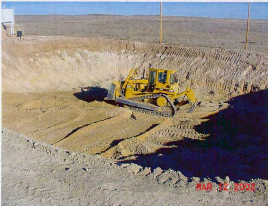
Top Photo: Pit 2 excavation, preparing bottom for liner.
