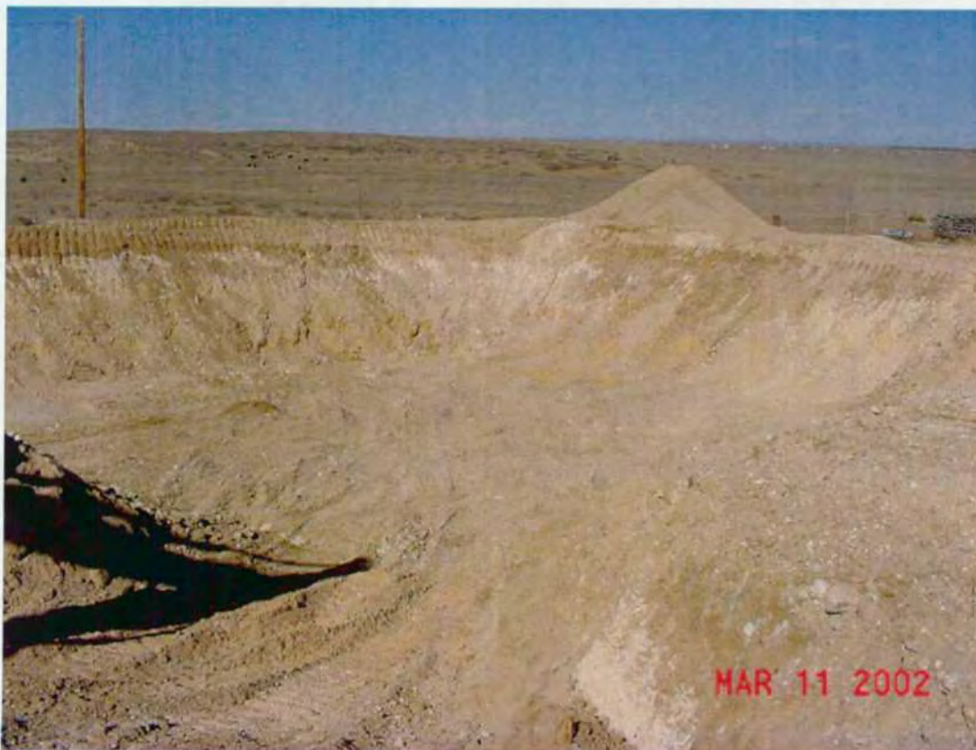
Bottom Photo: Pit 2 excavation complete.
