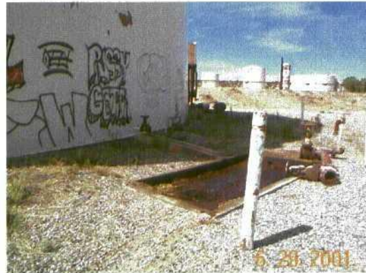
Pic #4- Far north 50000 bbl tank sump and sludge.
