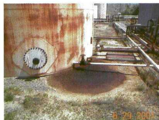
Pic # 12- Tank # 184 (or 18?). This tank was observed to have hydrocarbon product leaking from a valve and possibly under the tank.
