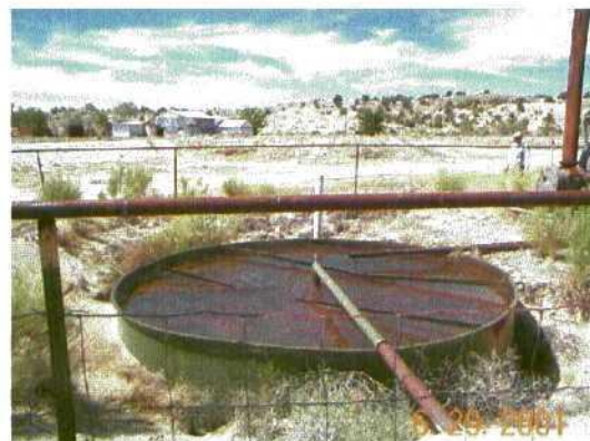
Pic #6- Buried produced water tank for on-site producing well.
