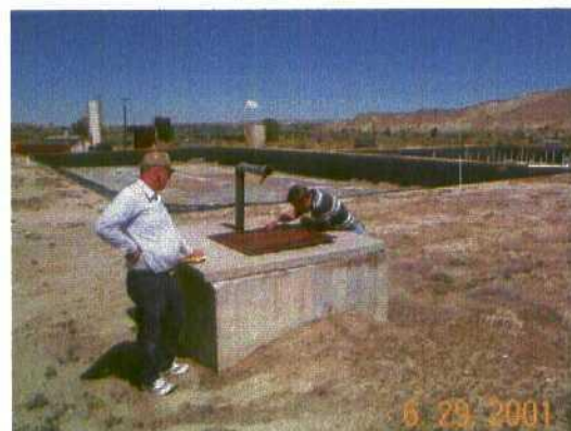
Pic #10 - Old plant main wastewater drain sump- Sump was noted to have fresh oil in it.
