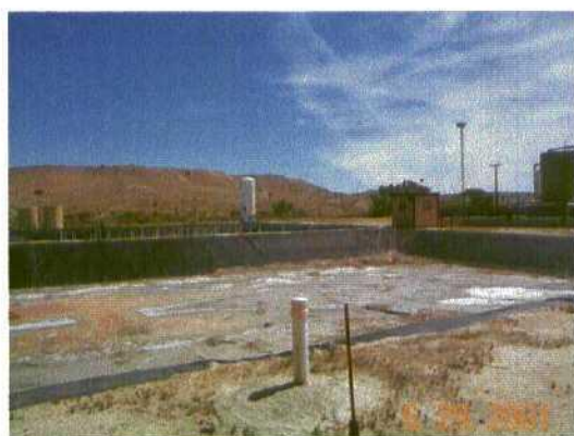
Pic # 9- Old plant waste water ponds and possible leak detectors.
