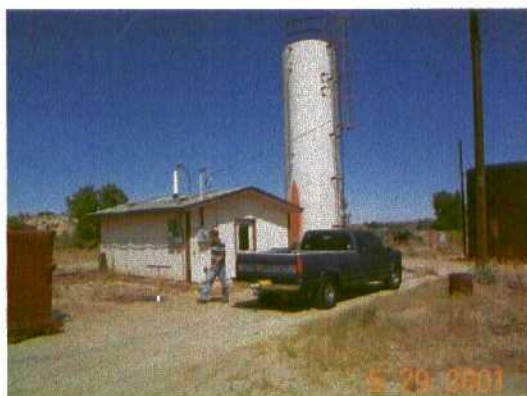
Pic #8- Far west side of plant area- Groundwater stripper tower.
