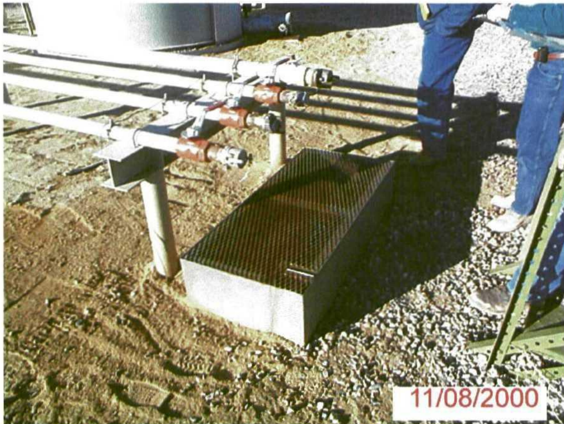
Picture #2- Tank farm single wall metal sump.
