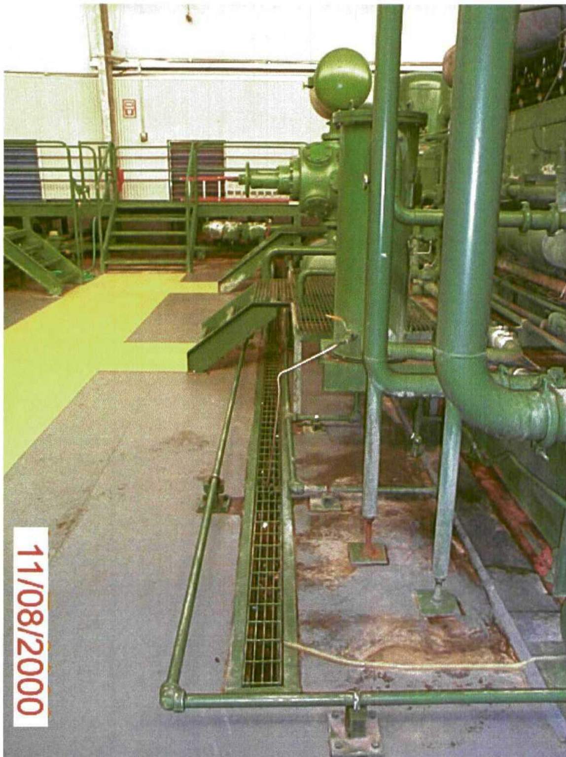
Picture #5- Floor drain troughs – typical of all compressor sites.
