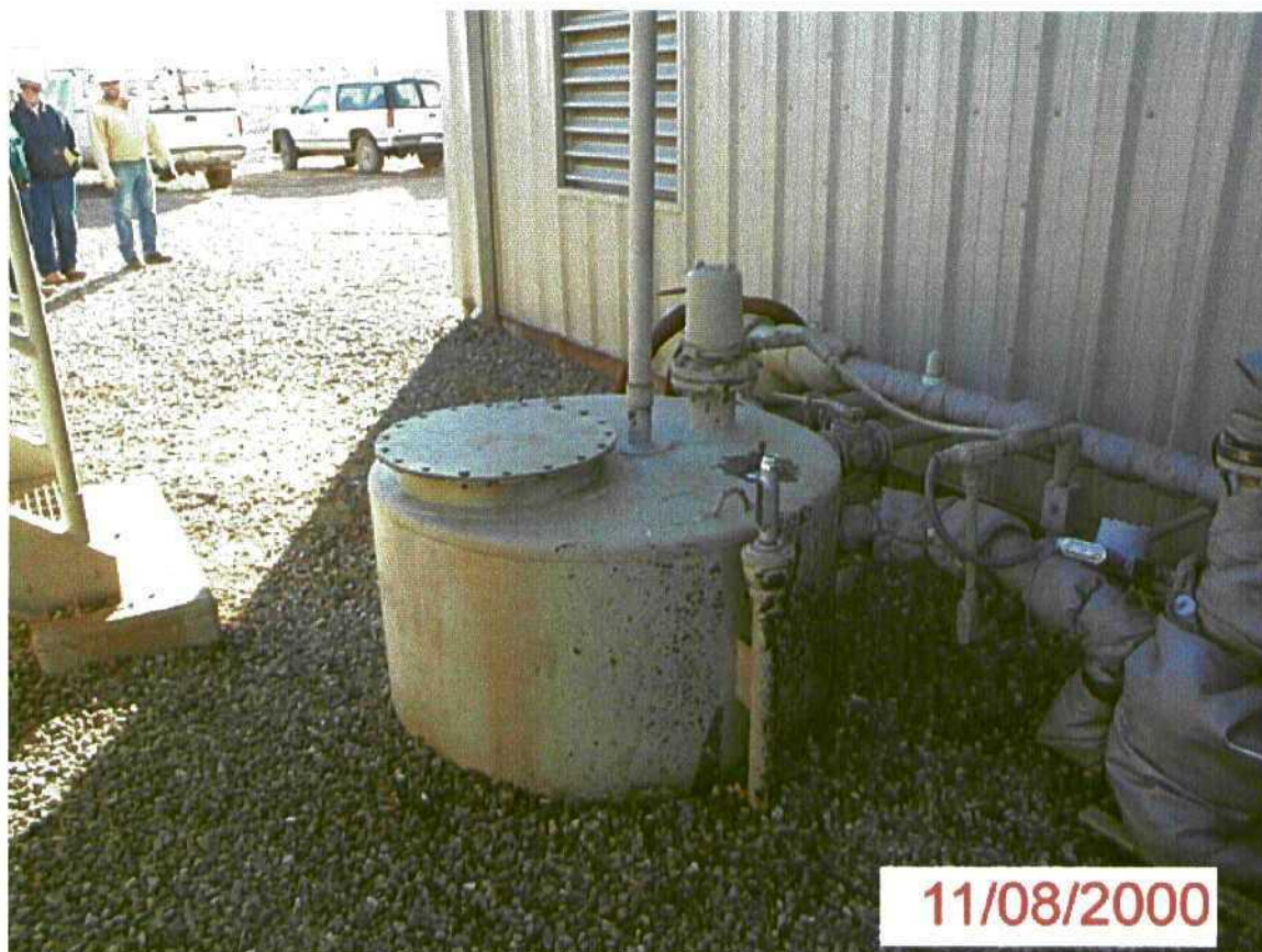
Picture #3- Main compressor sump- Burlington to investigate mechanical integrity of secondary system.
