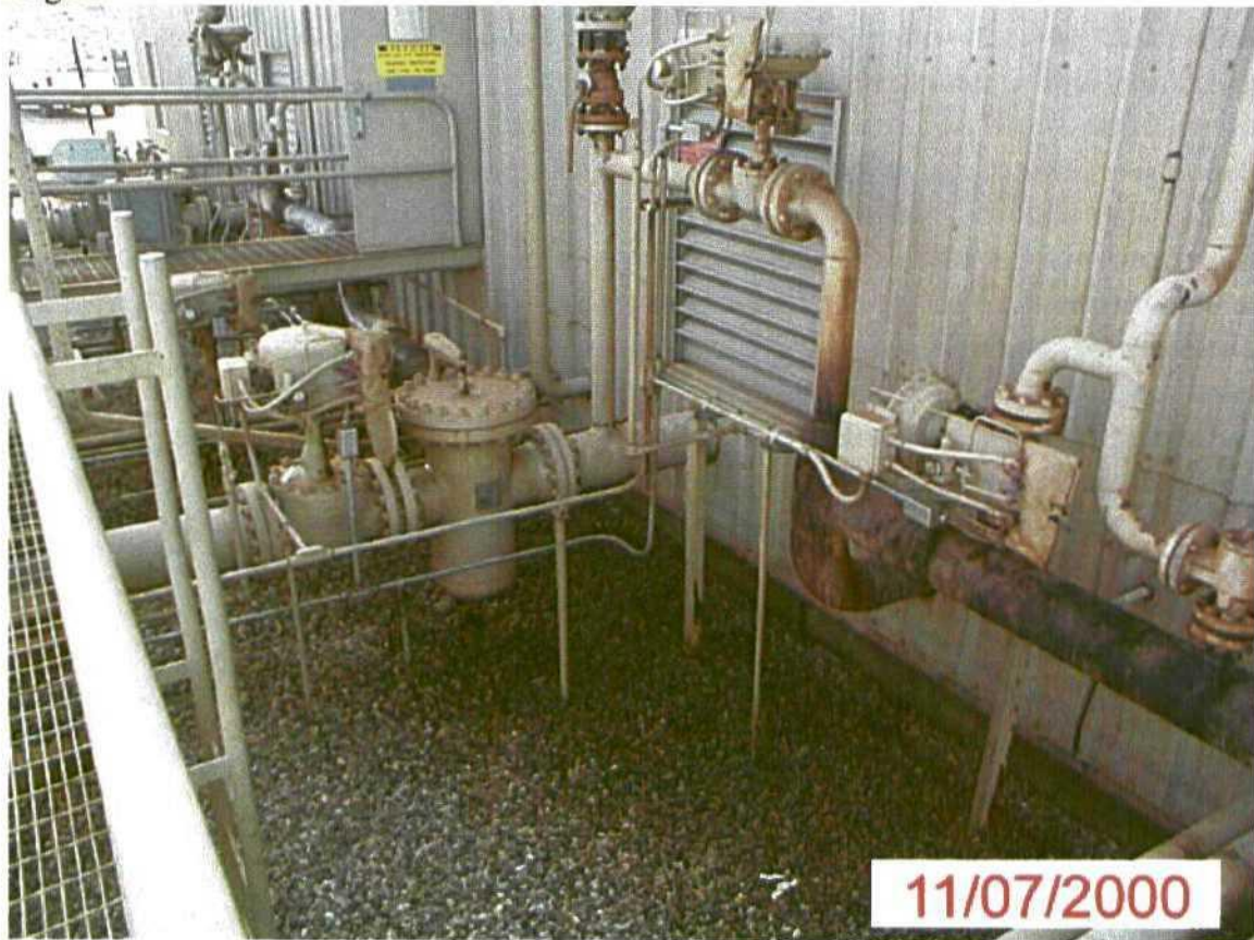
Picture #2- North side of Compressor Building oil stain from compressor stacks above.
