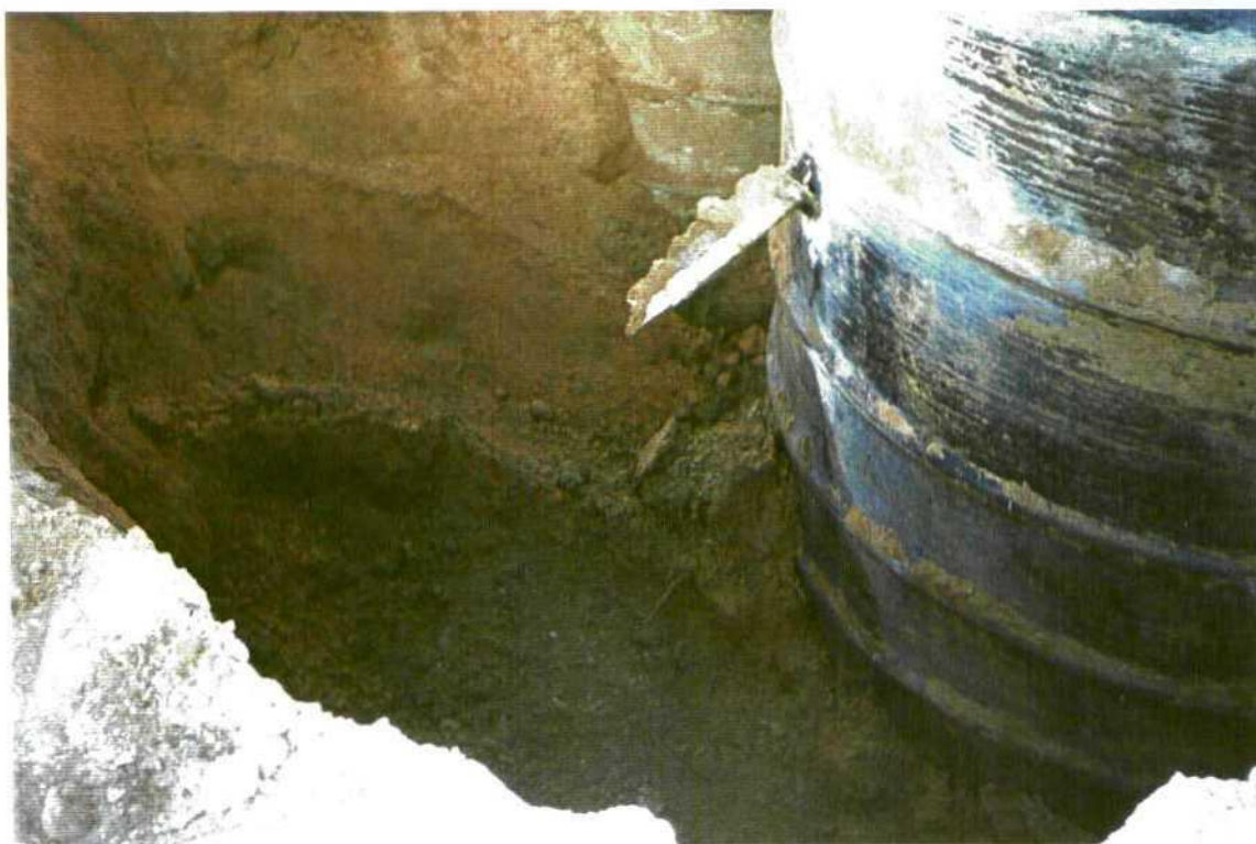
Photograph #7 Tank C showing piping juncture; Notice stain radiating down from piping juncture
