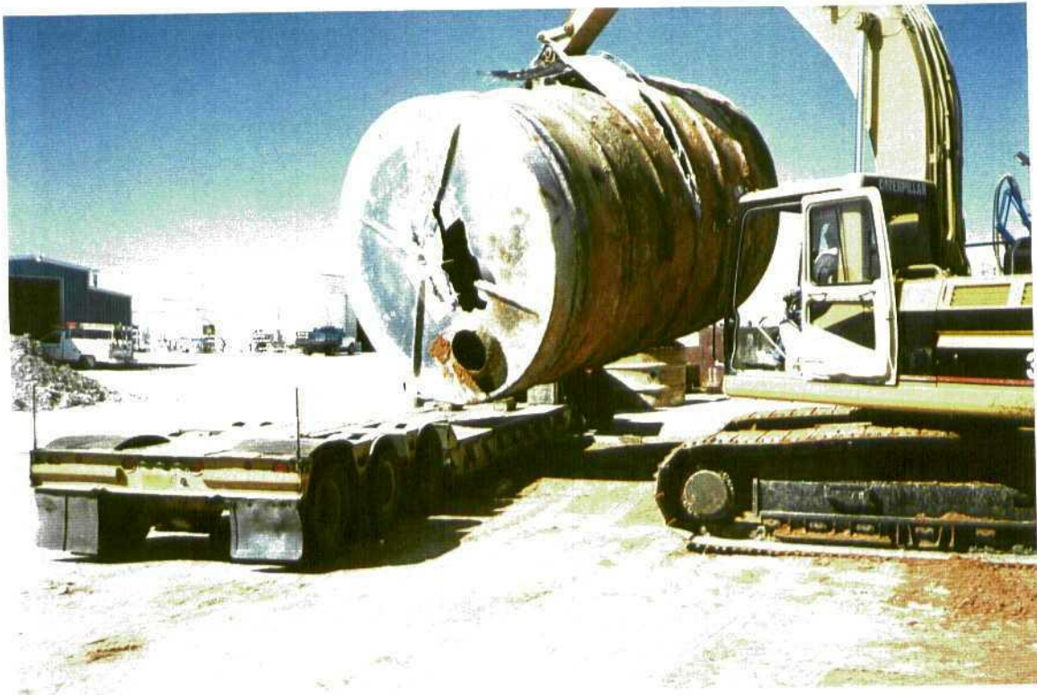
Photograph #11 Tank C being loaded onto trailer for transport to Rhino landfill (typical loading procedure)
