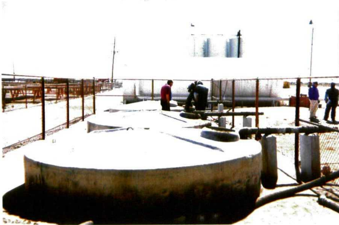
Date: 04/24/95 Picture Taken by: Lynette Collins, PRC Direction Facing: E Picture Description: Underground gravity separation Tanks A, B, and C, located east of the Sand Trap Tank
