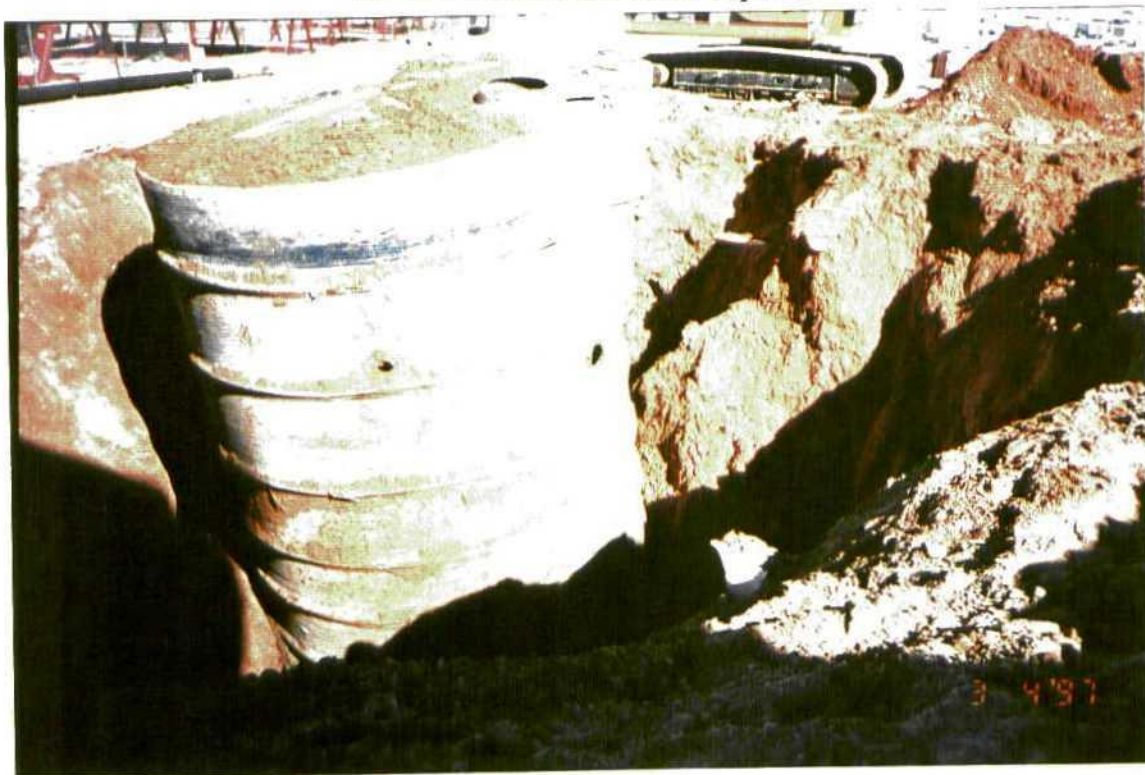
Photograph #6 Three large wastewater tanks exposed; 800 gallon tank removed
