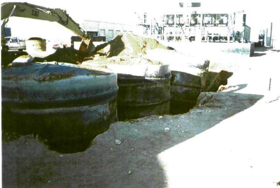
Photograph #5 All four wastewater tanks exposed
