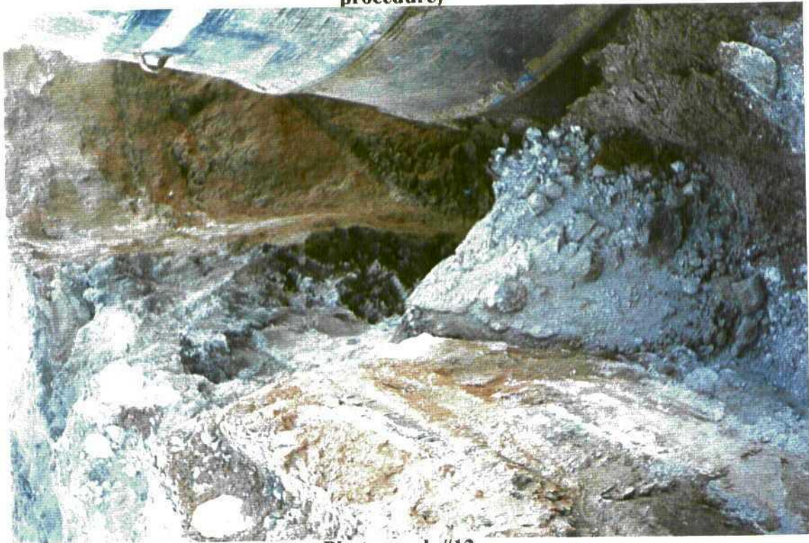
Photograph #12 Stained soil on east sidewall next to Tank D (near piping juncture)
