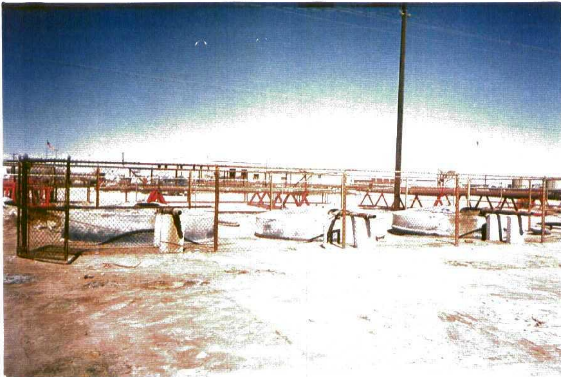
Photograph #1 Three 12,000 gallon wastewater tanks prior to removal
