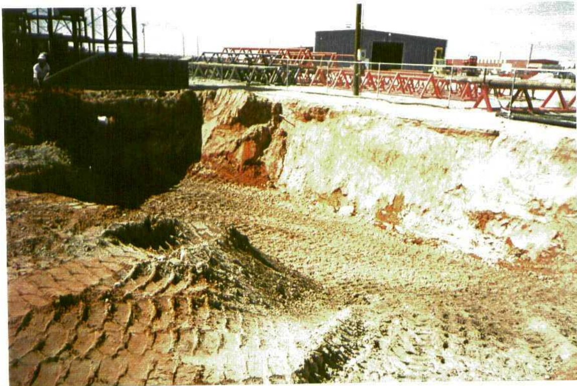
Photograph #20 Tank excavation partially backfilled
