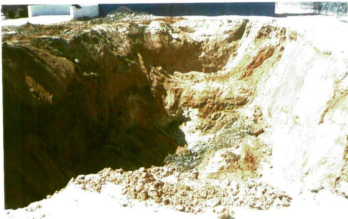
Photograph #15 Tank pit facing west wall after overexcavation (deepest point = 22 feet)
