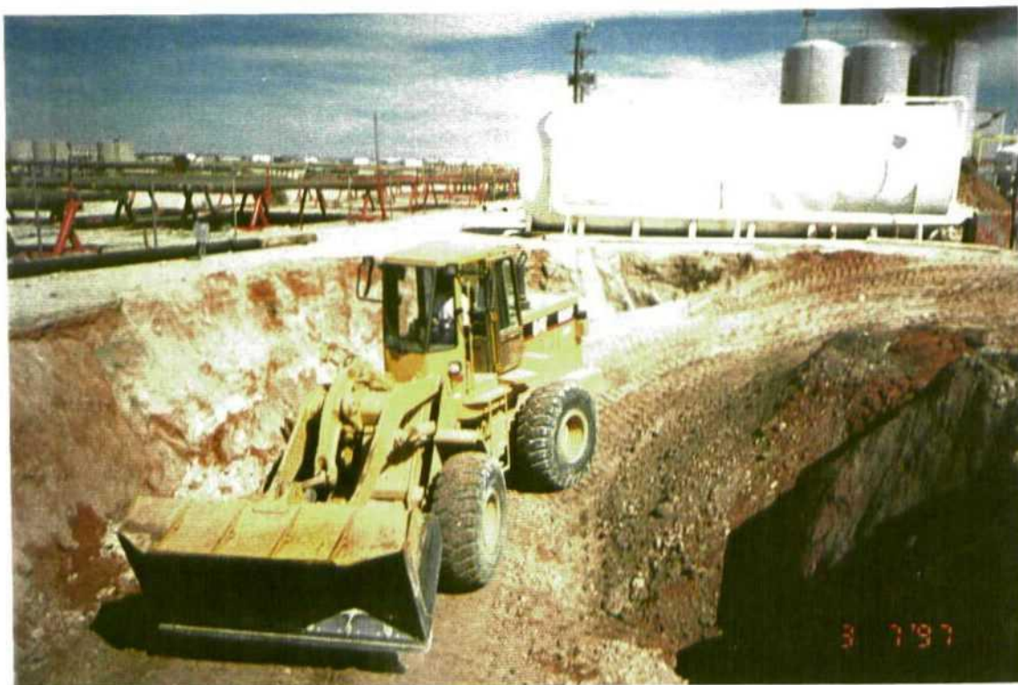
Photograph #21 Backfilling excavation
