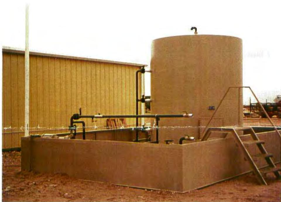
Photo 1: Diesel/Polymer Storage Vessel
