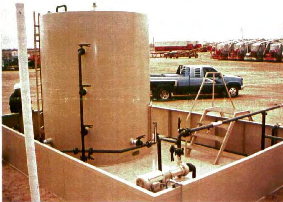
Photo 2: Vessel's Secondary Containment
