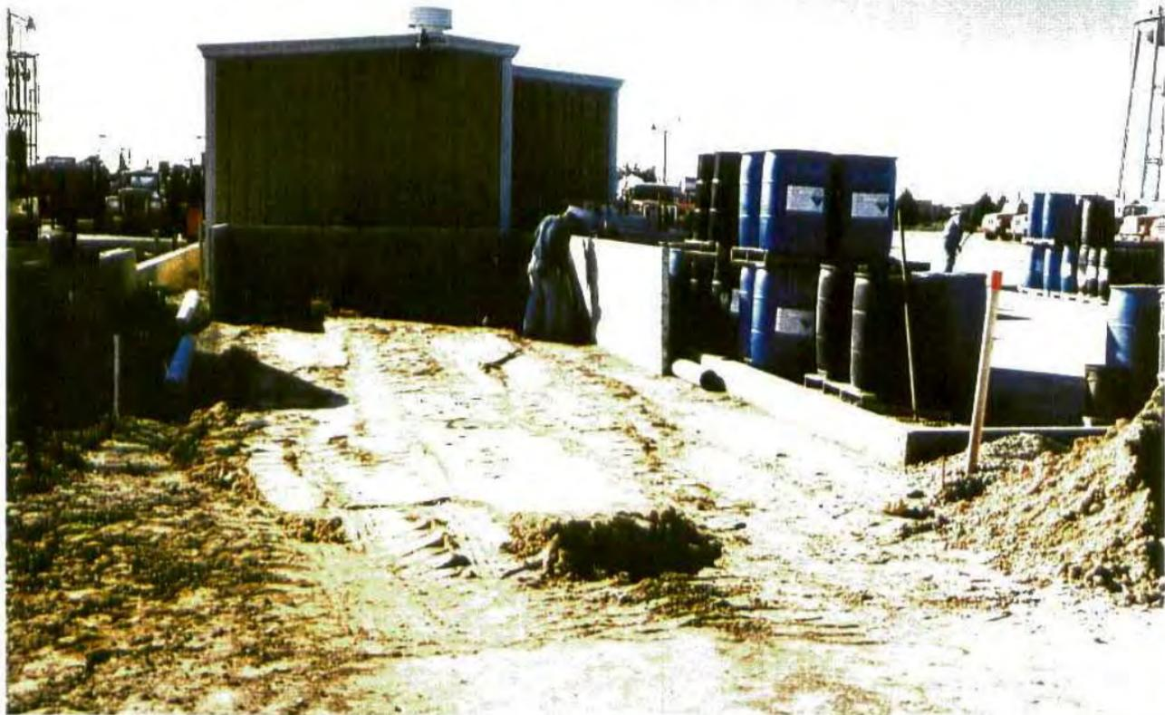
LINER SECURED AT TOP OF WALL FOR HCl ACID STORAGE
