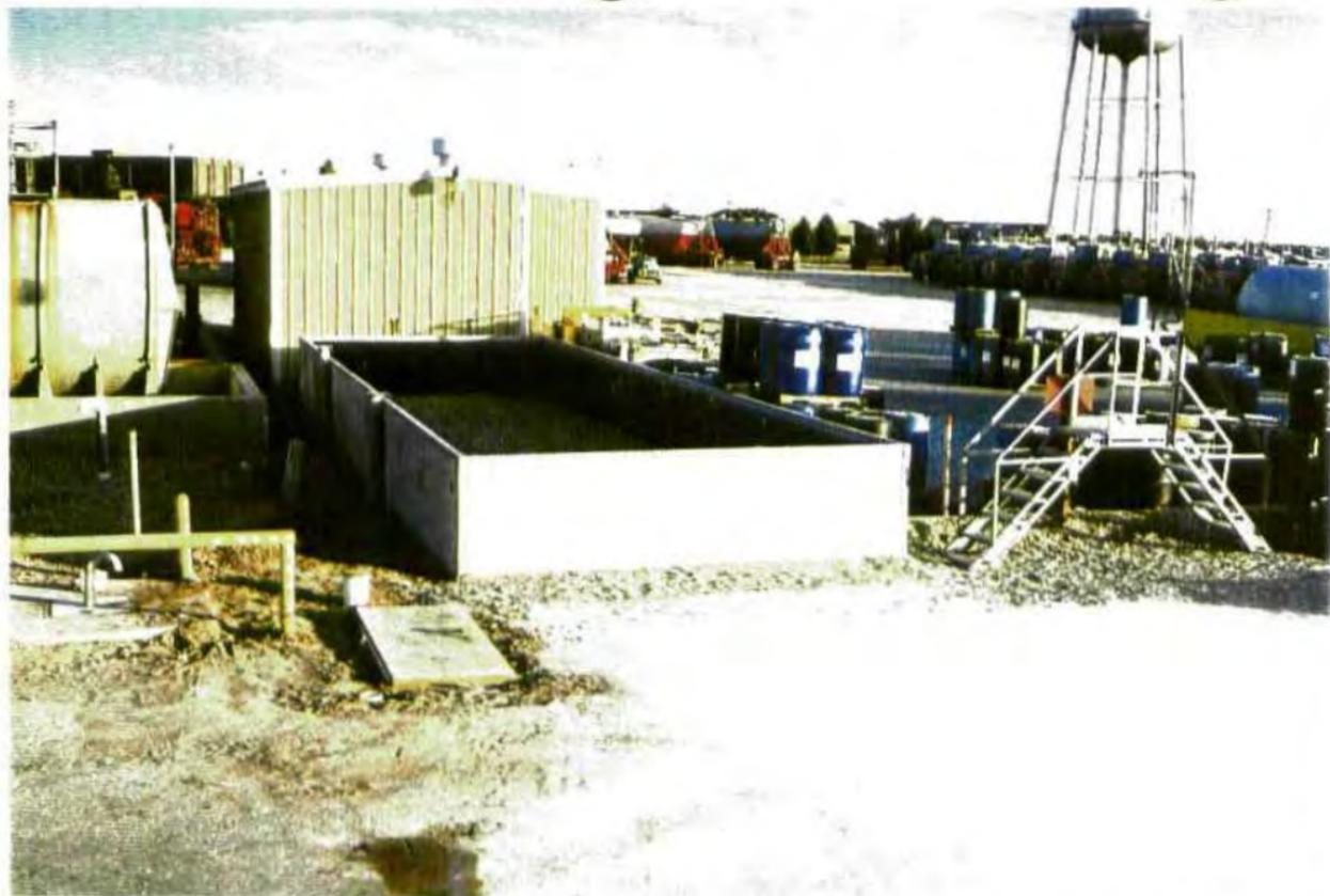
LINER SECURED AT TOP OF WALL FOR HCl ACID STORAGE
