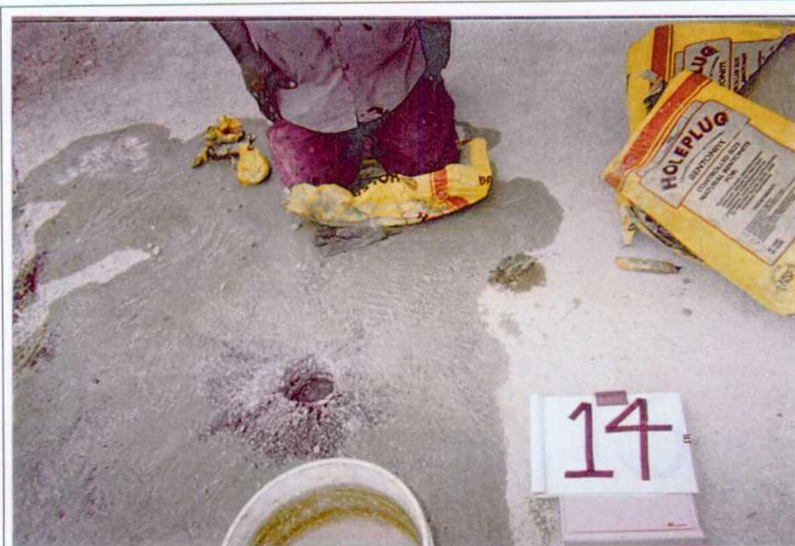
14. Driller plugging W3IB.
