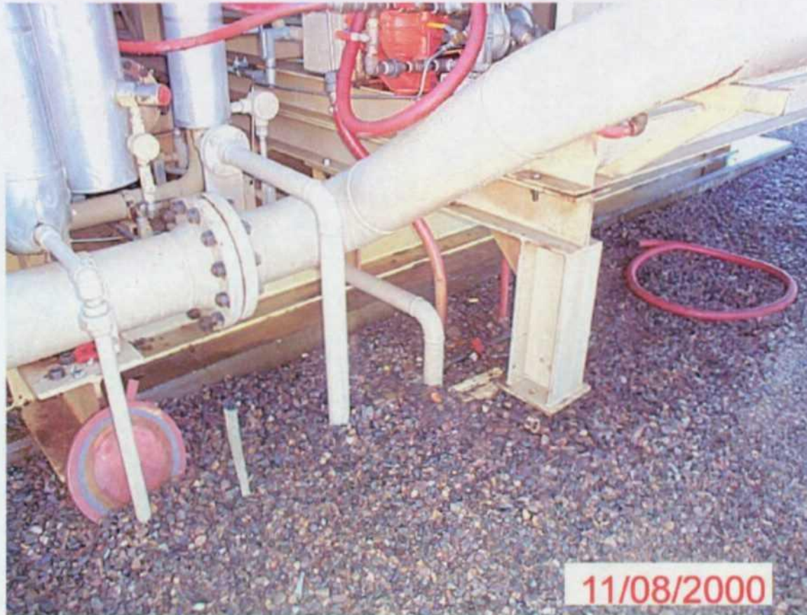
Picture #3- West side (outside) Compressor oil and water discharge to ground.
