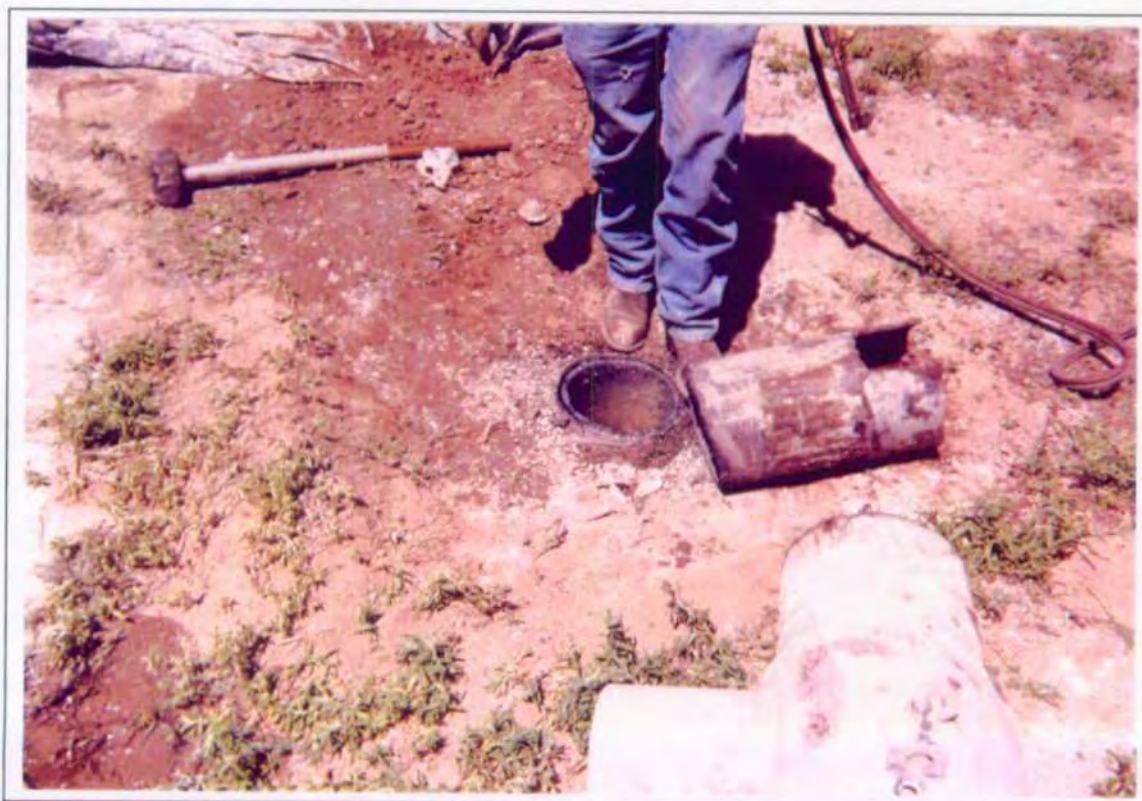
Cement Shoe; 9-3/4" Casing in Monitor Well 6-3 10-3/4" Casing
