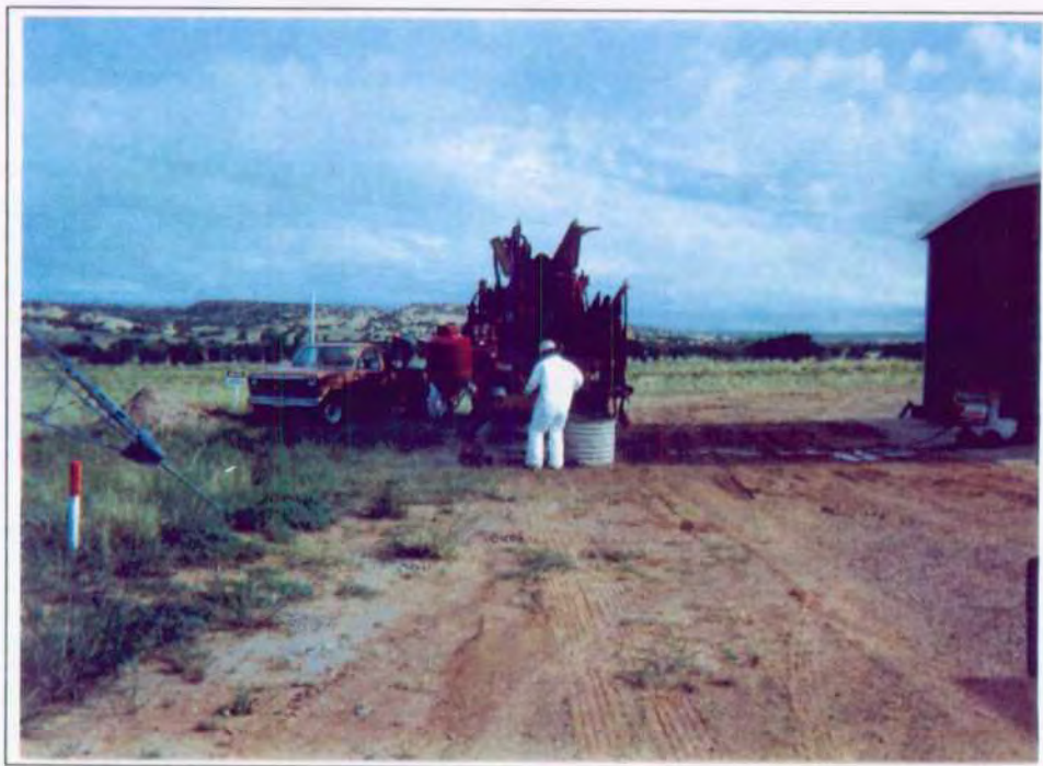
Steam Cleaning Pipe Truck Tools and Bits Prior to Each Abandonment
