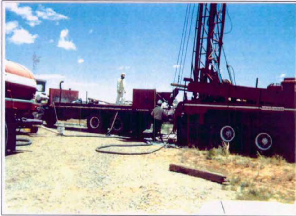
Typical Cementing Operation
