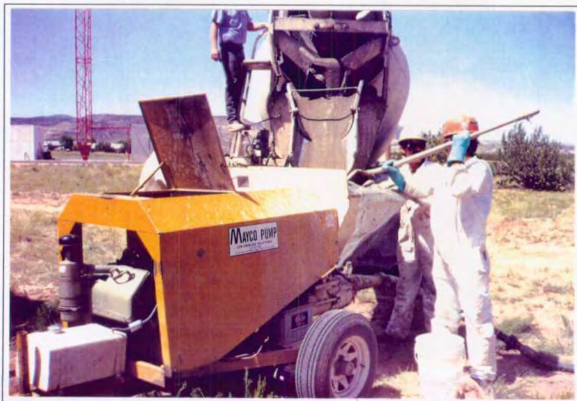
Mixing and Pumping Cement
