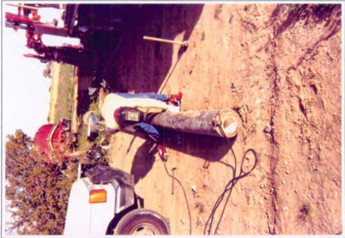
Welding Cement Shoe to 9-3/4" Casing
