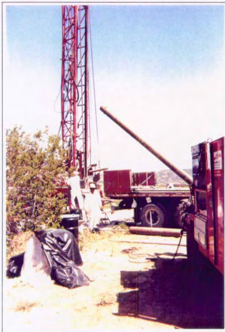
Re-Drilling Monitor Well 6-3
