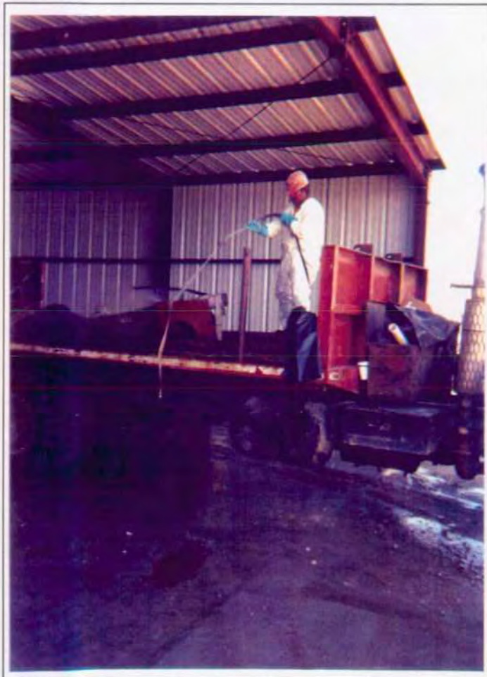
Steam Cleaning Pipe Truck Tools and Bits Prior to Each Abandonment
