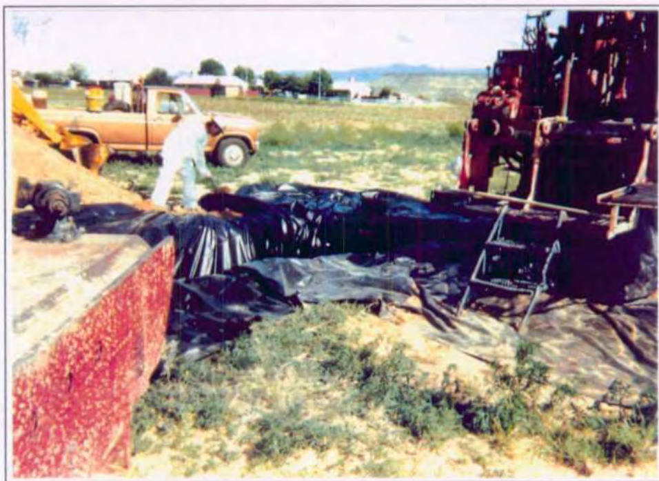
Digging and Lining Mud Pit on Monitor Well 6-2
