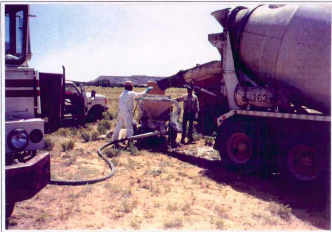
Cementing Monitor Well 6-2
