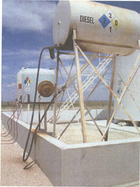
Image 2: Saddle tanks within secondary containment area. Tanks might need to be moved back and away from edge of curbing. Worst case scenario of breached hose or valve on tank will lead to discharge on to the ground.
