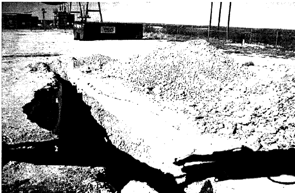
The edges of the pits were identified by exposing a plastic liner under a caliche cap.
