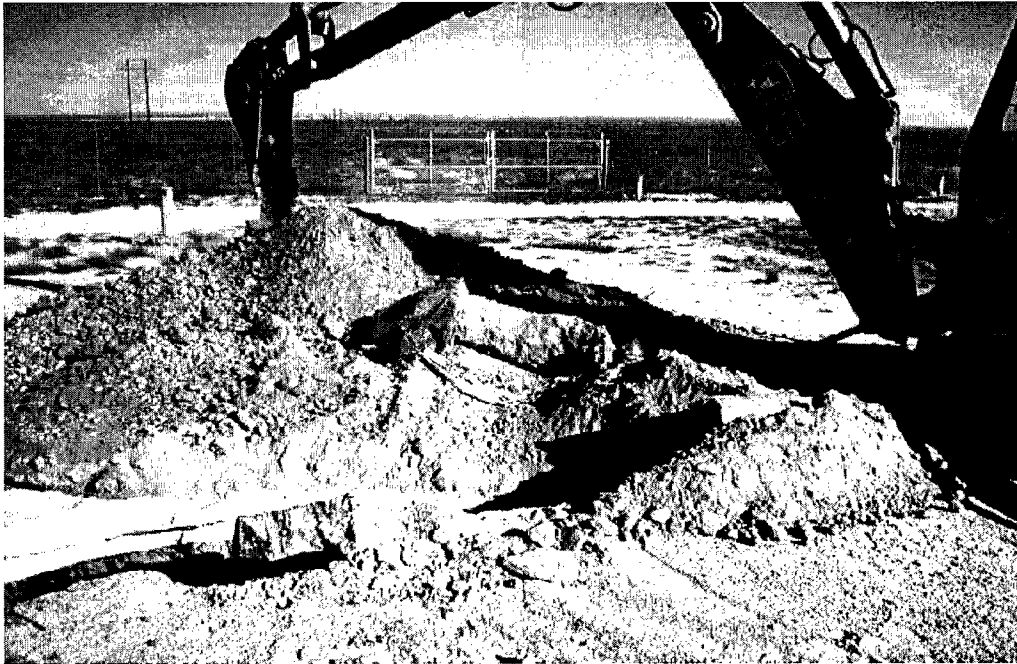
Excavation of a trench for collecting soil samples in the Engine Room Drain Pit Area.
