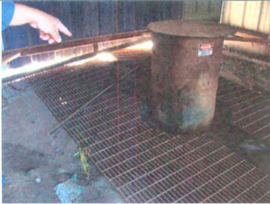
Photo 11: 1 of 3 below grade tanks associated with wash area.
