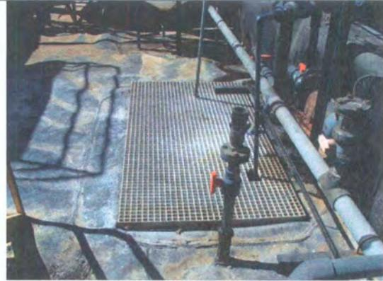
Photo 4: Below grade tank within a lined bermed area.
