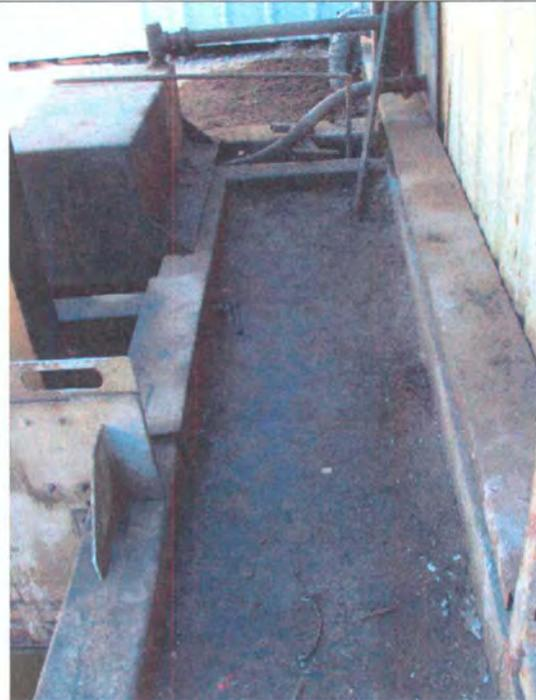
Photo 9: Soil staining around fluids holding area
