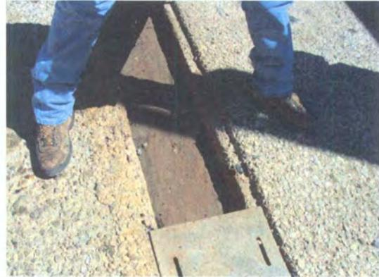
Photo 10: Sediments in wash bay area drainage system.
