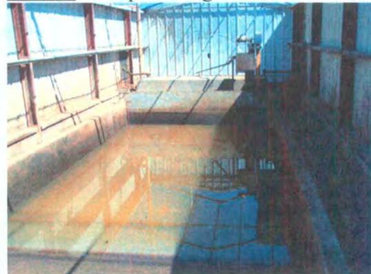
Photo 6: Wash bay effluent in holding tank.
