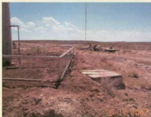
Wastewater tank, different view. Berming needs work. Yates will address and send pictures when work is complete.
