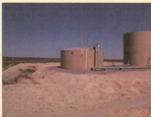
Other tanks at same site showing proper berming and housekeeping.
