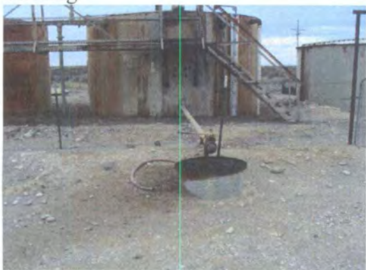
Photo 9: Catch pan with discharge on ground.
