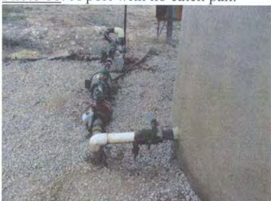
Photo 12: Contamination around an unlined AST.
