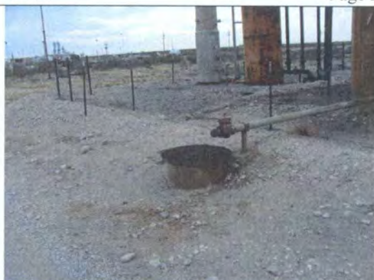
Photo 10: Second catch pan with soil staining.
