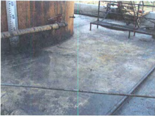
Photo 2: More cracks in secondary containment.
