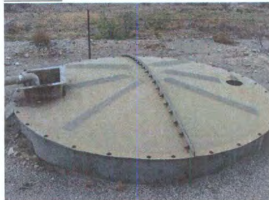
Photo 15: One of two below grade tanks without proper containment.
