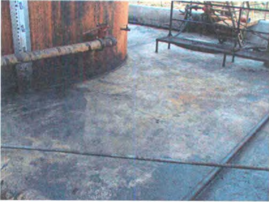
Photo 2: More cracks in secondary containment.
