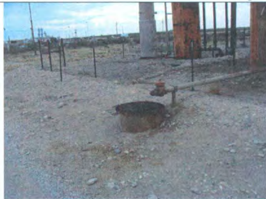
Photo 10: Second catch pan with soil staining.
