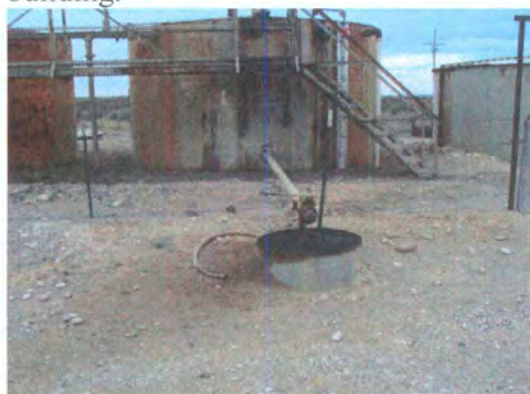
Photo 9: Catch pan with discharge on ground.
