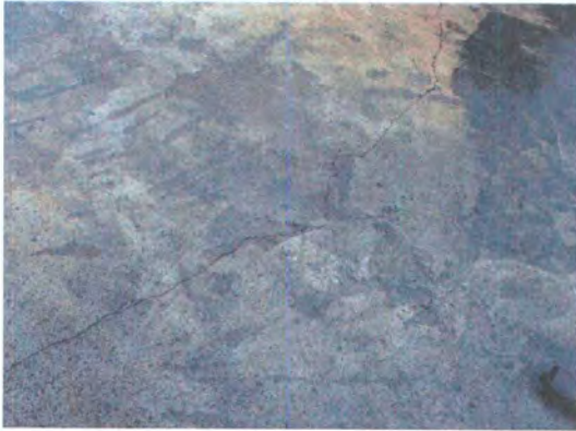
Photo 1: Crack in a concrete secondary containment.
