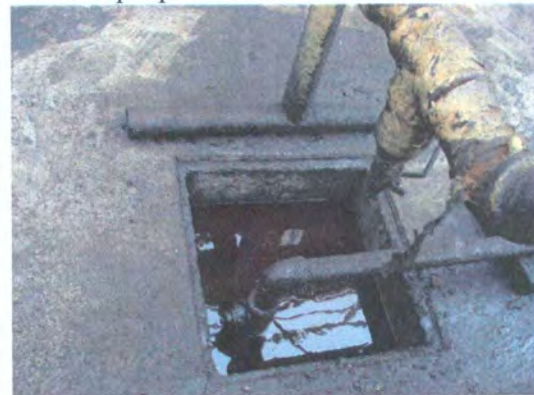
Photo 17: Sumps being used as below ground tanks.
