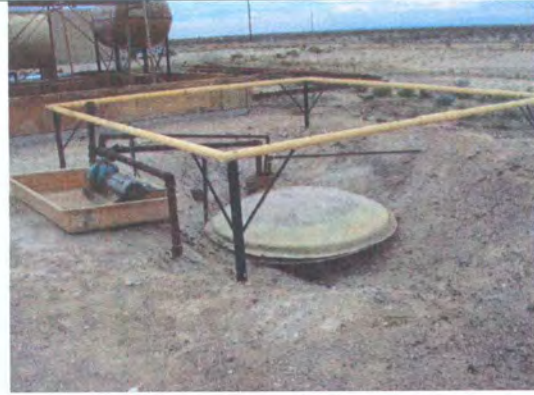
Photo 16: Two of two below grade tanks without proper containment.
