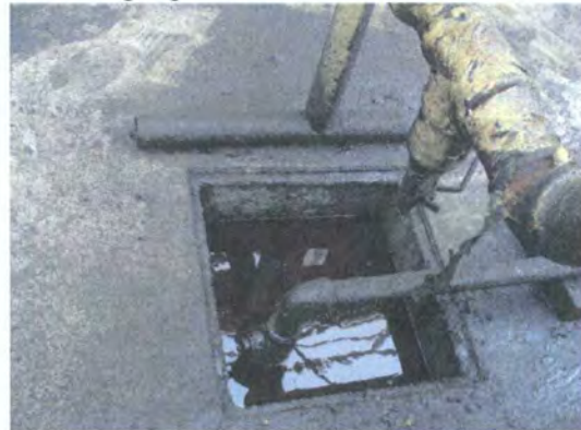
Photo 17: Sumps being used as below ground tanks.
