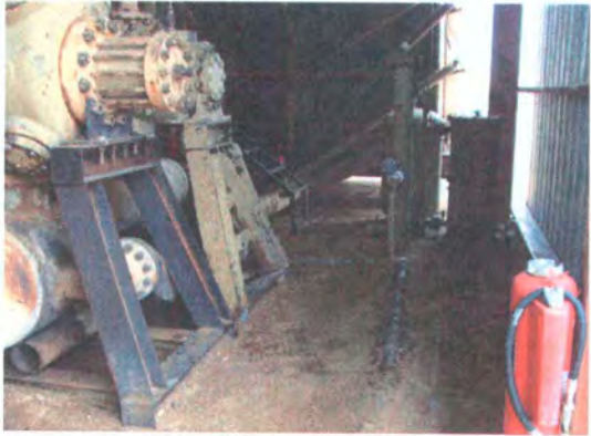
Photo 6: Contaminated soil near compressor.
