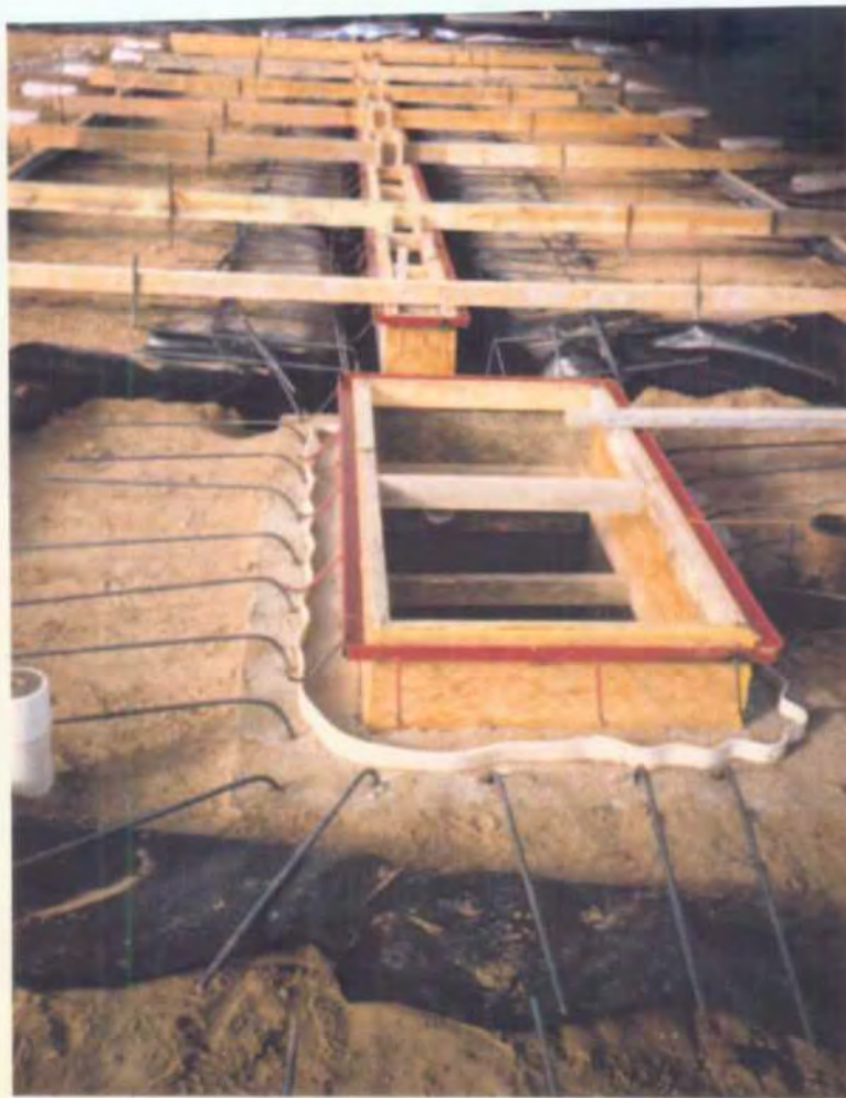
Formed and lined floor drain and sump
