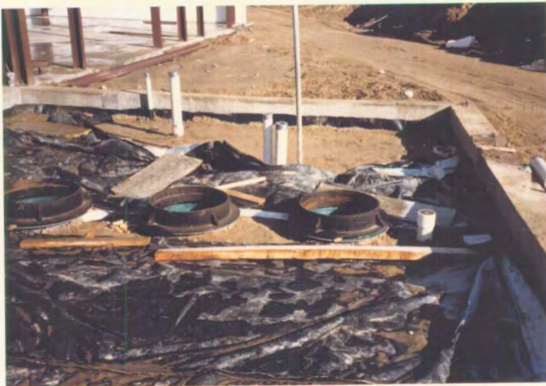
Separator installed with leak detection system
