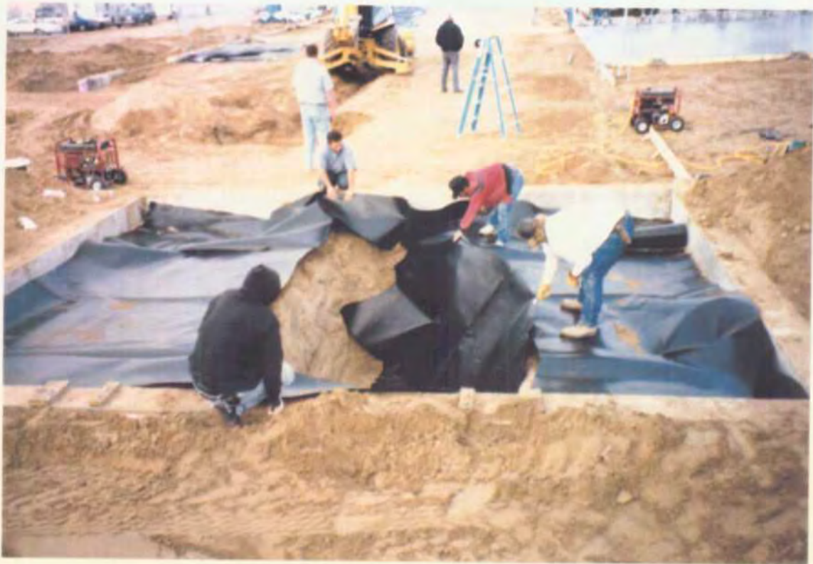
Installation of HDPE liner in separator excavation
