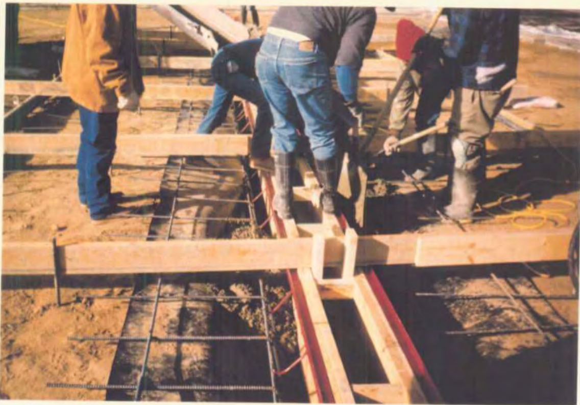
Pouring concrete around floor drain (note HDPE liner below concrete)
