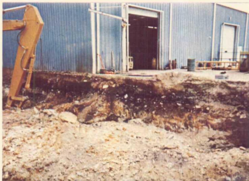
A-14. Contamination Along South Wall of Area A Excavation
