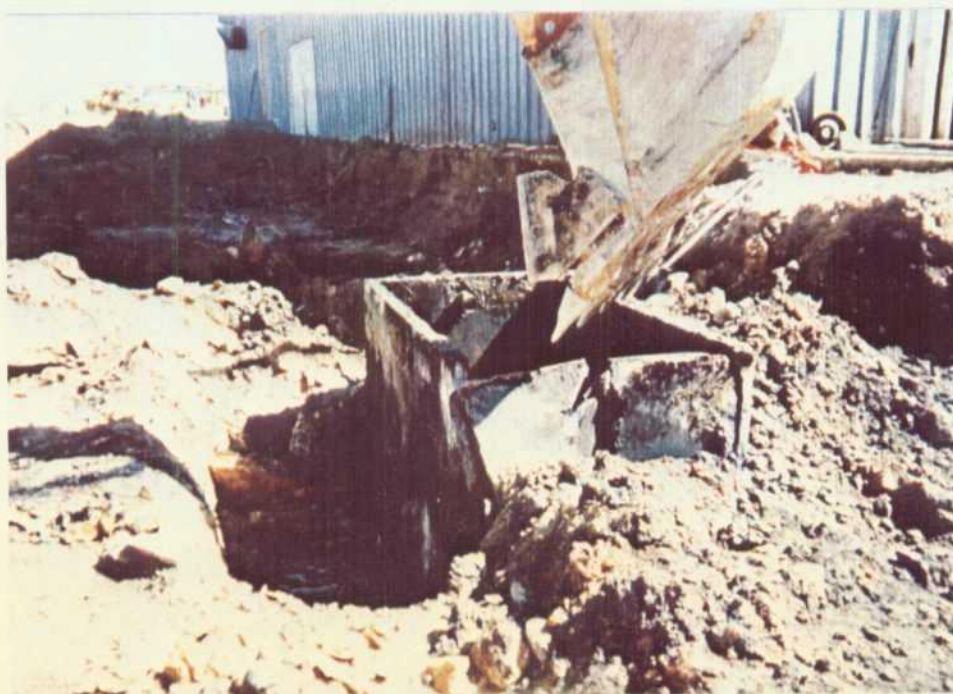
A-11. Removal of HFTO Building's Holding Tank
