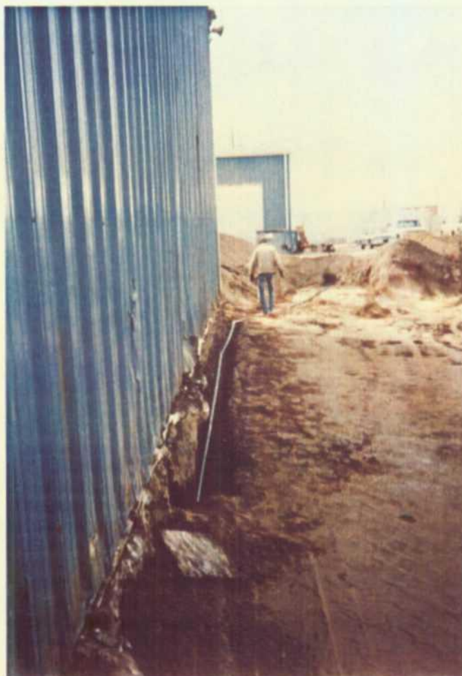
A-19. Transfer Line Between HWS Sump and HFTO Building's Oil/Water Separator
