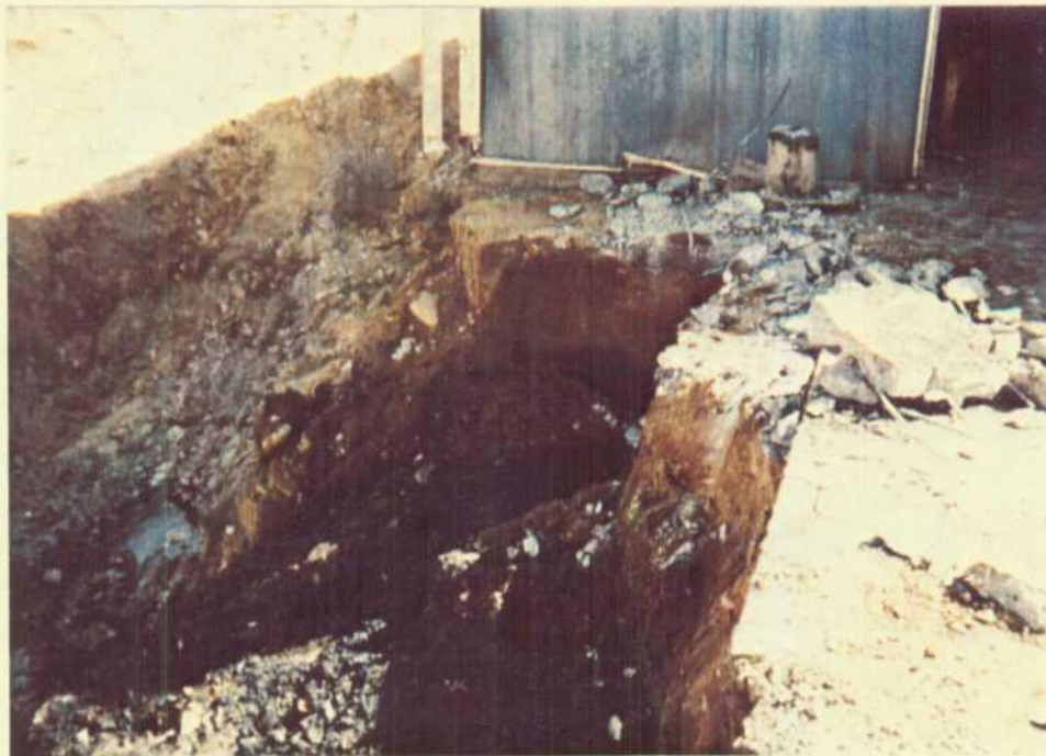
A-16. Damage to HFTO Building After Sump Removal
