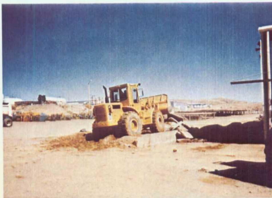
A-7. Demolition of HFTO Building's Concrete Pads
