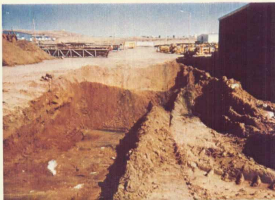
A-8. Stained Soils Exposed from Underneath HFTO Buildings's Concrete Pads
