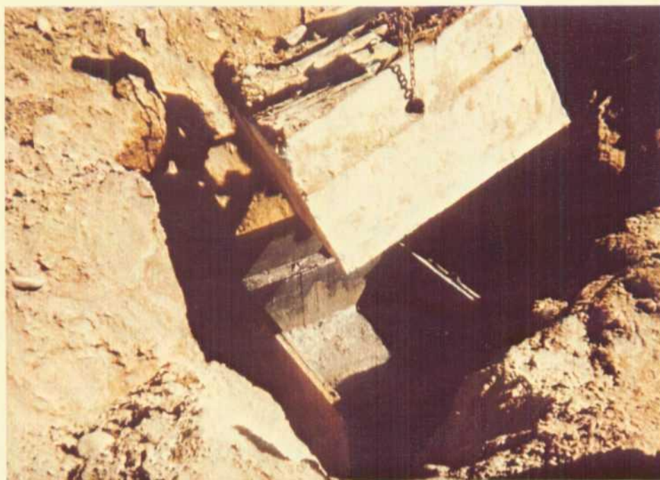
A-6. Removal of Top Half of HWS Building's Holding Tank
