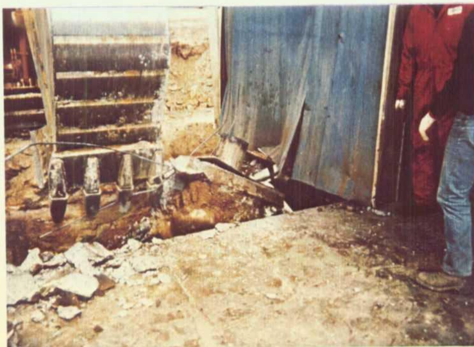
A-17. Damage to HFTO Building After Removal of the Base of the Crane
