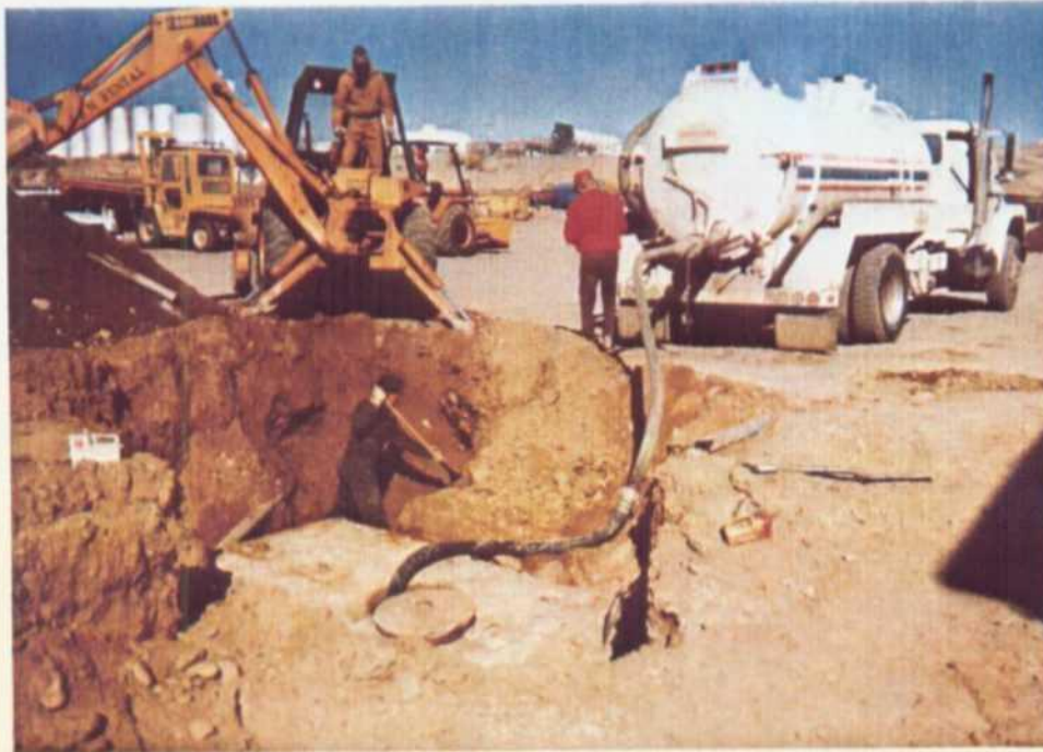
A-3. Transferring HWS Building's Holding Tank Water to Truck
