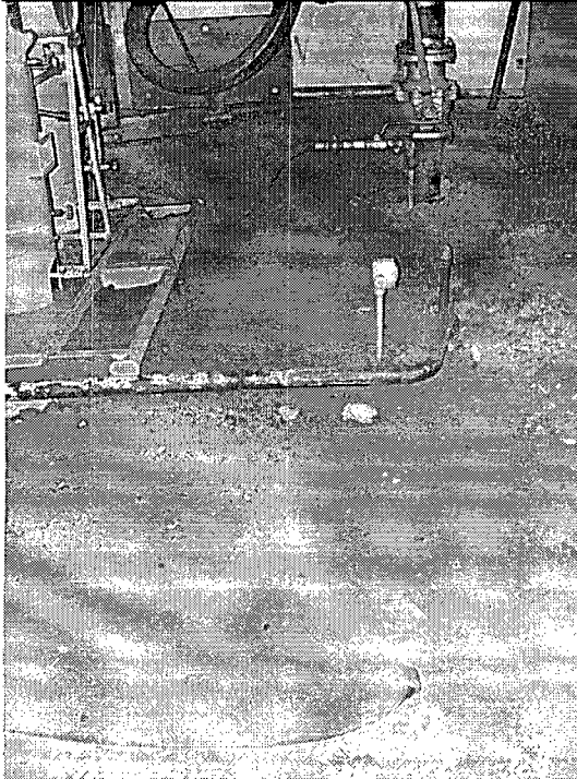
Photo 6: Soil contamination around engine.
