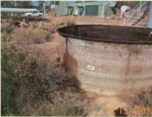
7. Fiberglass open top tank has oil and water in it. Tank is leaking waste onto ground.
