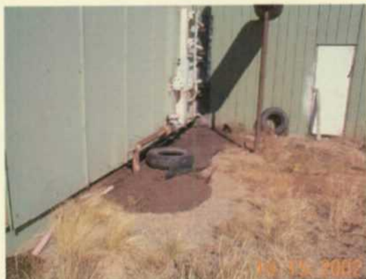
2. Oil discharged to ground near compressor air inlet.
