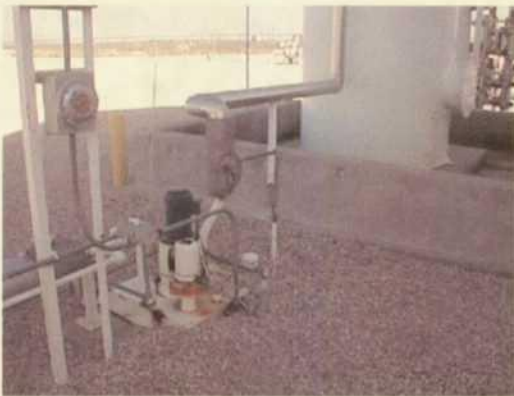
East side turbine drain sump-has secondary containment.
