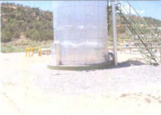
Photo 7: Conoco Phillips tank without appropriate liner.
