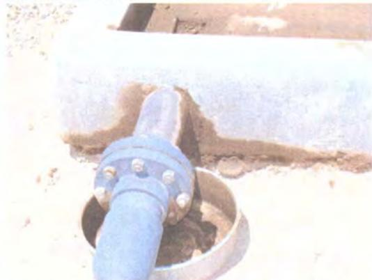
Photo 5: Same as photo 4 close up of cracks on the edge.
