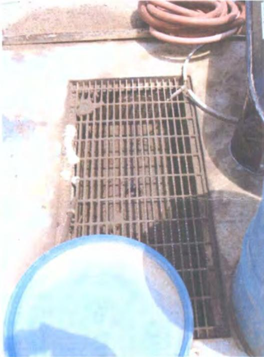
Photo 1: Sump with residual oil stains.
