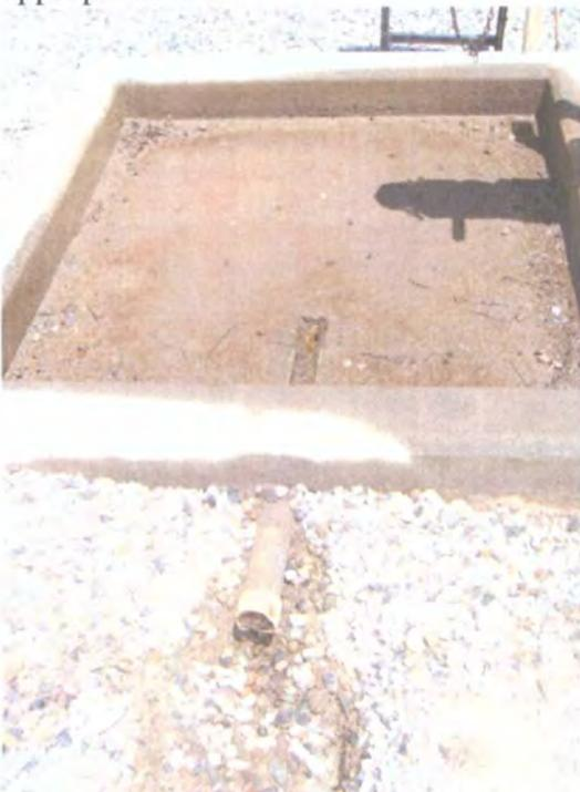
Photo 8: Unused secondary containment with residual discharge on to ground.
