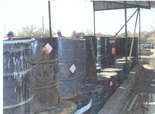
Photo 4: Barrels stacked within containment.
