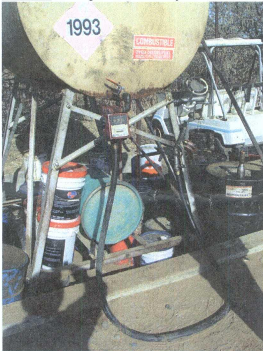
Photo 2: Saddle tank for diesel fuel.
