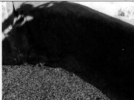
Photo 10: A hole in a secondary containment liner.
