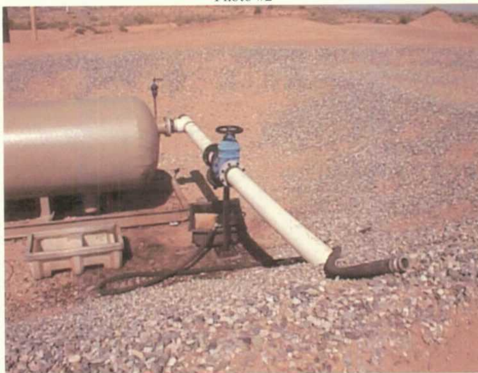
GW-045 WILLIAMS FIELD SERVICES KUTZ CANYON GAS PLANT Leak/spill onto ground surface at oil/water separator July 7, 1999
