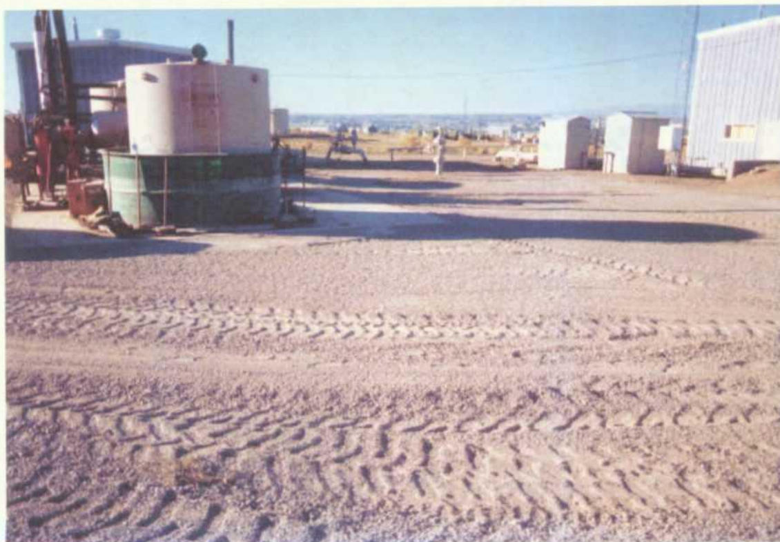
Photo #6 - East side of concrete slab, excavation, complete, gravel replaced, view west
