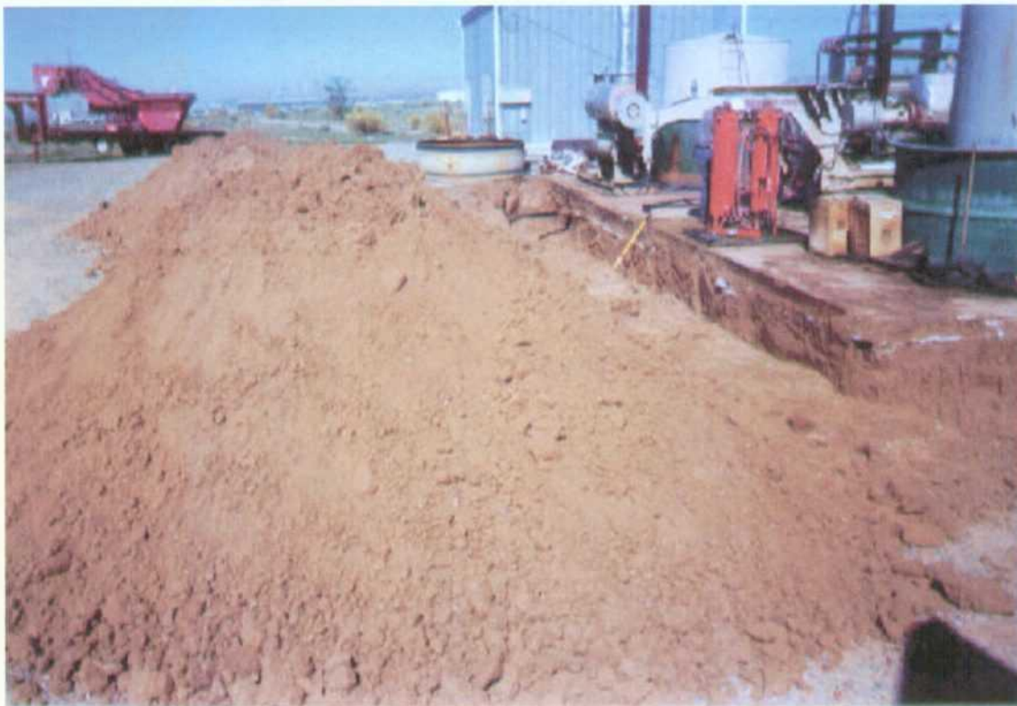
Photo #12 - South side of concrete slab, excavation complete, gravel replaced
