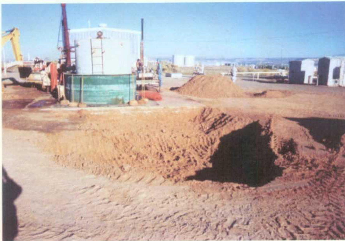
Photo #6 - East side of concrete slab, excavation, complete, gravel replaced, view west
