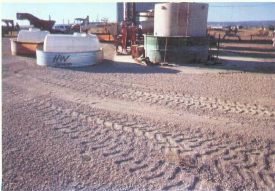
Photo #12 - South side of concrete slab, excavation complete, gravel replaced
