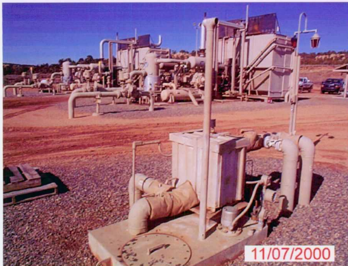
Picture #2- Main Sump with Leak detection
