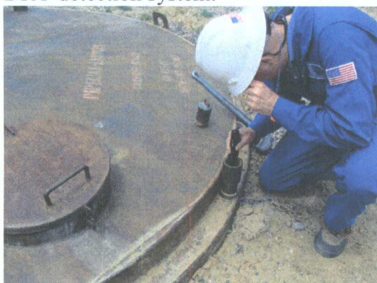
Photo 9: 2 of 3 BGT on-site, verified DRY detection system.
