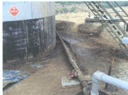
Photo 5: Discharge of unused tank.
