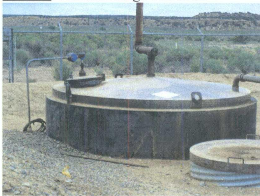
Photo 8: 1 of 3 BGT on-site, verified DRY detection system.
