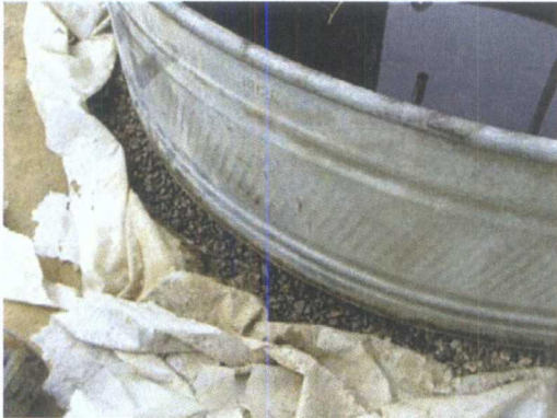
Photo 13: Containment in photo 12 appears to have seepage of contents.
