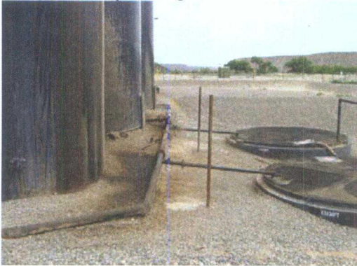
Photo 2: BGT's behind unlined AST's where spill occurred. GW impacted, as of inspection monitored only but not remediated.
