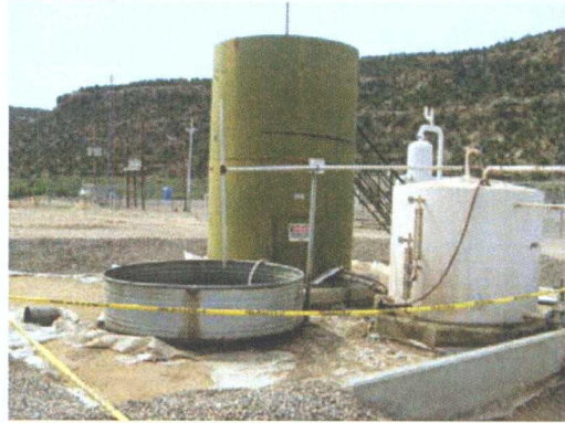
Photo 5: AST's with deteriorated lining.
