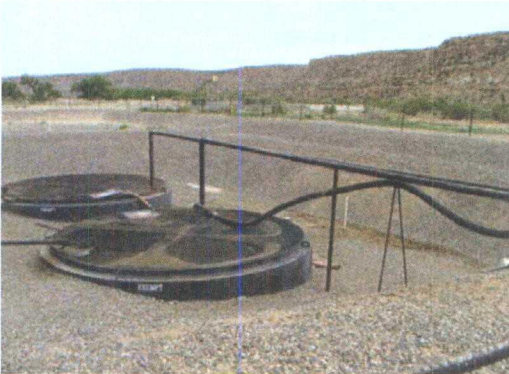
Photo 3: Leak detection of one BGT has fluids the other BGT could not verify leak detection system due to un-removable port.
