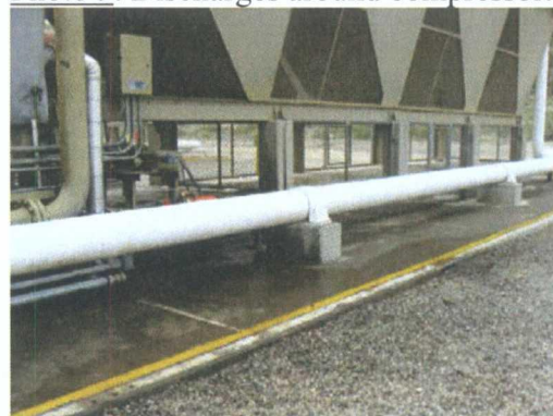
Photo 10: Discharges near compressor.
