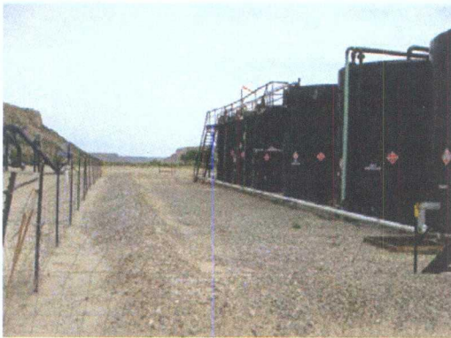
Photo 1: Unlined AST's where spill occurred 1.5 years ago.
