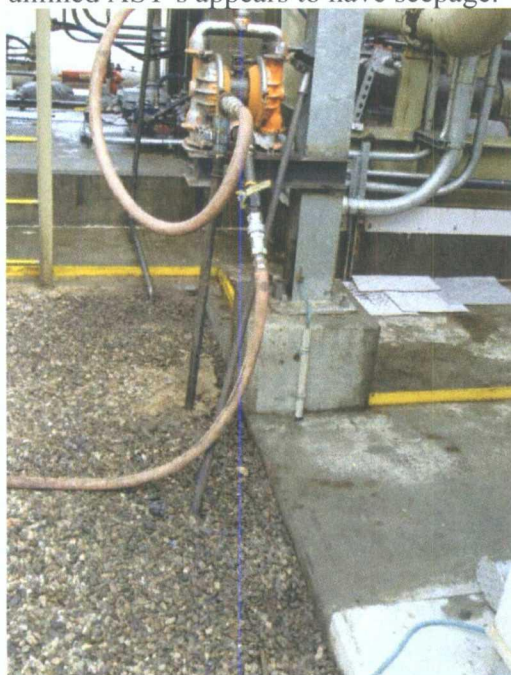
Photo 8: Around compressor have discharges on to ground.
