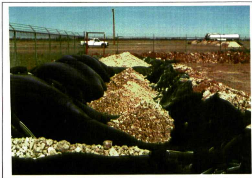
Photo No. 2. Stockpiled excavated soil from leach field pit.
