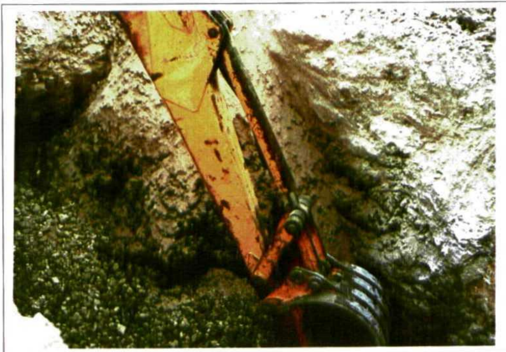
Photo No. 5. Excavation of hydrocarbon stained gravels (black) from leach field collection pit.
