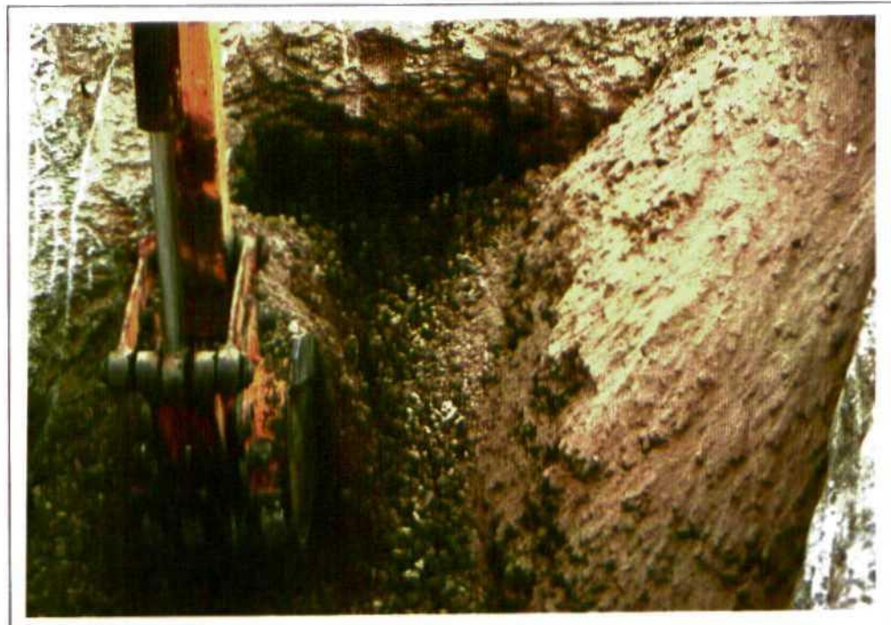
Photo No. 6. Excavation of Hydrocarbon contaminated gravels (black) from leach field collection pit.
