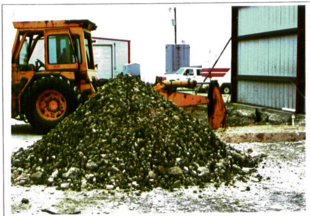
Photo No. 3. Excavation of leach field pit. Note hydrocarbon stained gravels.
