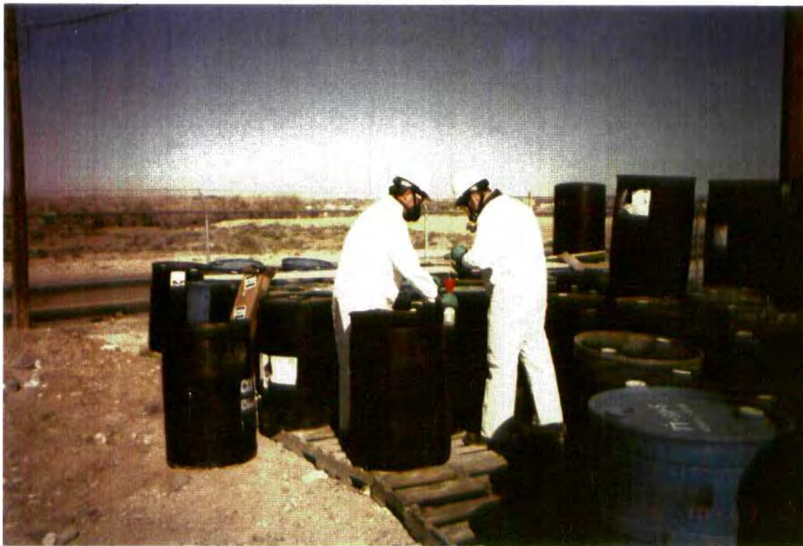
Date: 04/05/95 Picture Taken by: Luis Vega, PRC Direction Facing: NW Picture Description: PRC collecting sample CDI-DR33-02 from Drum 33
