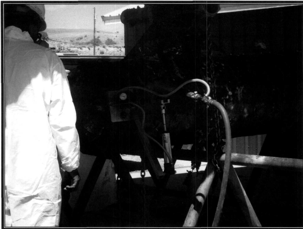
Photo 5: Line Drip Cutting Process
