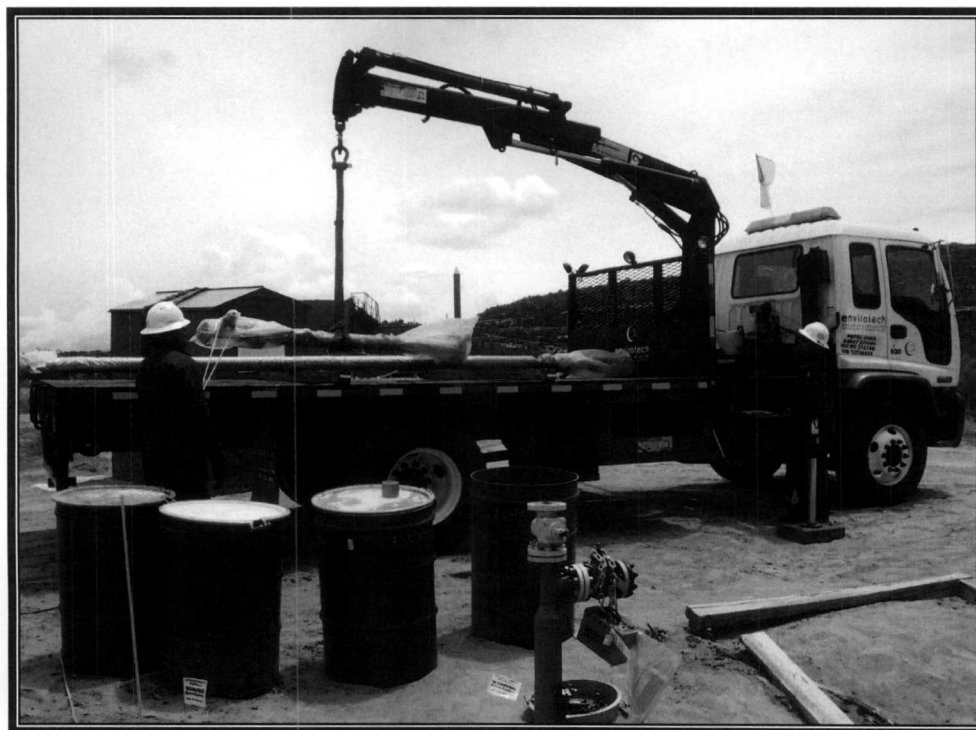
Photo 6: Loading Meter-Run and Tubing for Transportation
