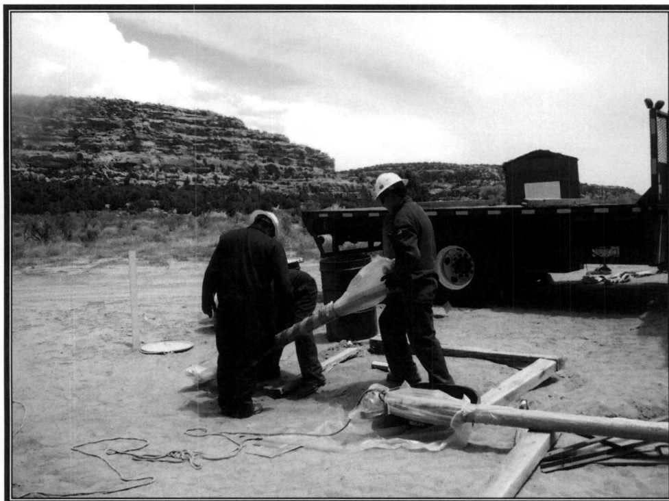
Photo 5: Preparing Meter-Run and Tubing for Transportation
