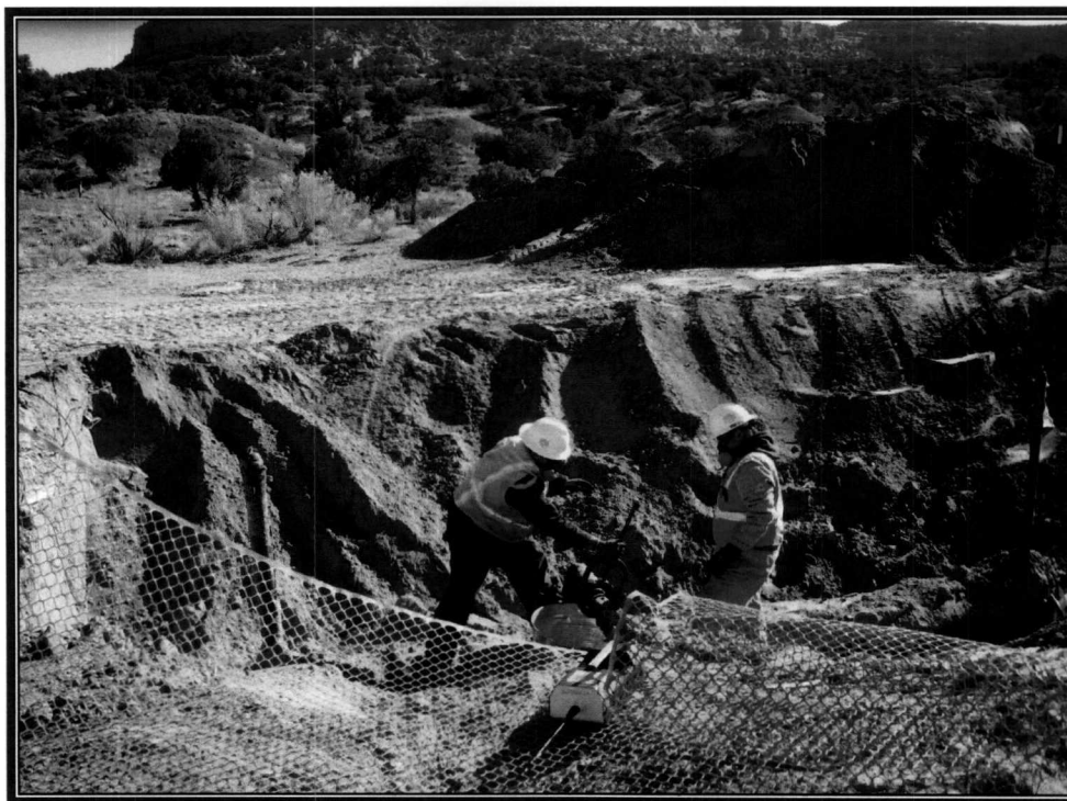
Photo 8: Cold Cutting Piping for Line Drip Removal (View 1)
