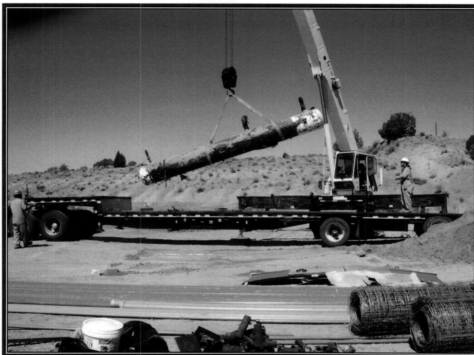
Photo 10: Loading Line Drip for Transportation
