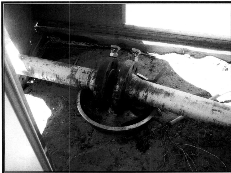
Photo 2: Meter Run Disassembly (View 1)
