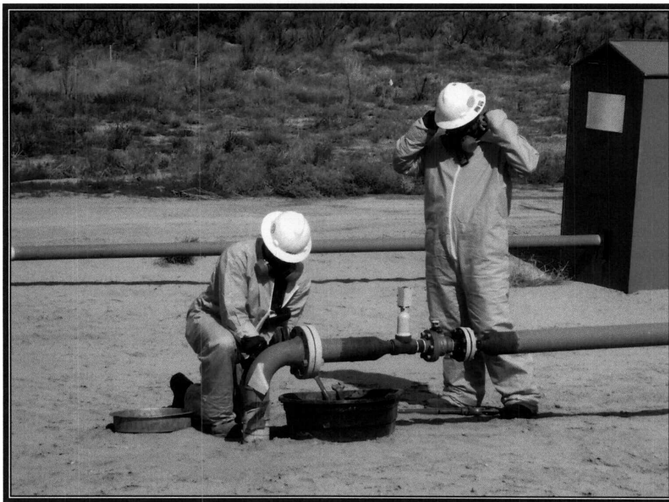
Photo 4: Meter Run Disassembly (View 3)
