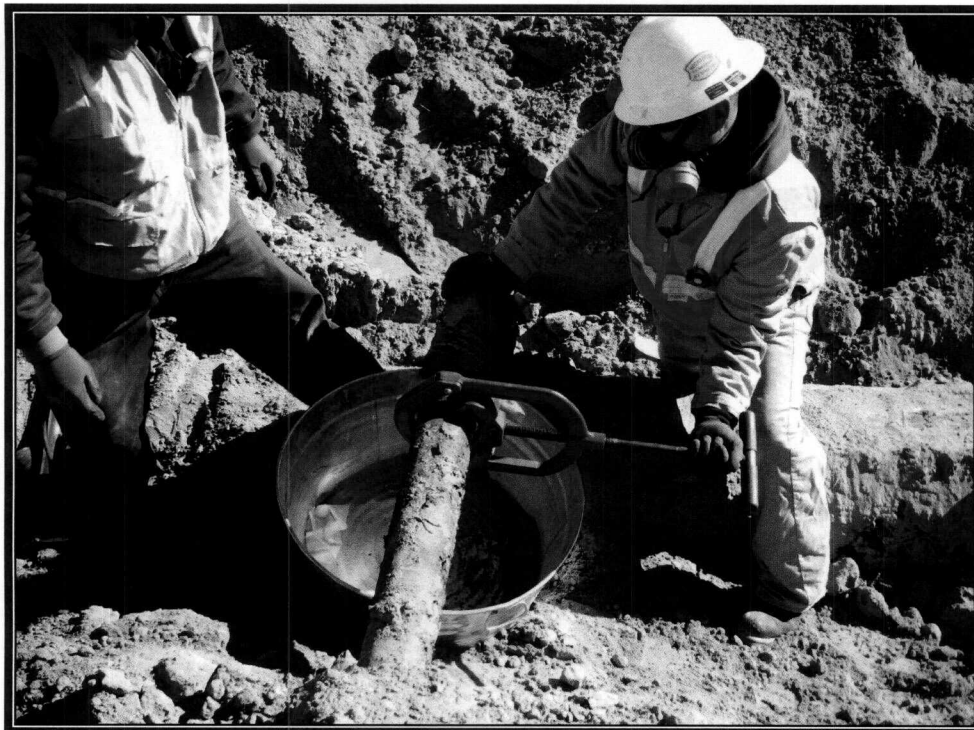
Photo 9: Cold Cutting Piping for Line Drip Removal (View 2)
