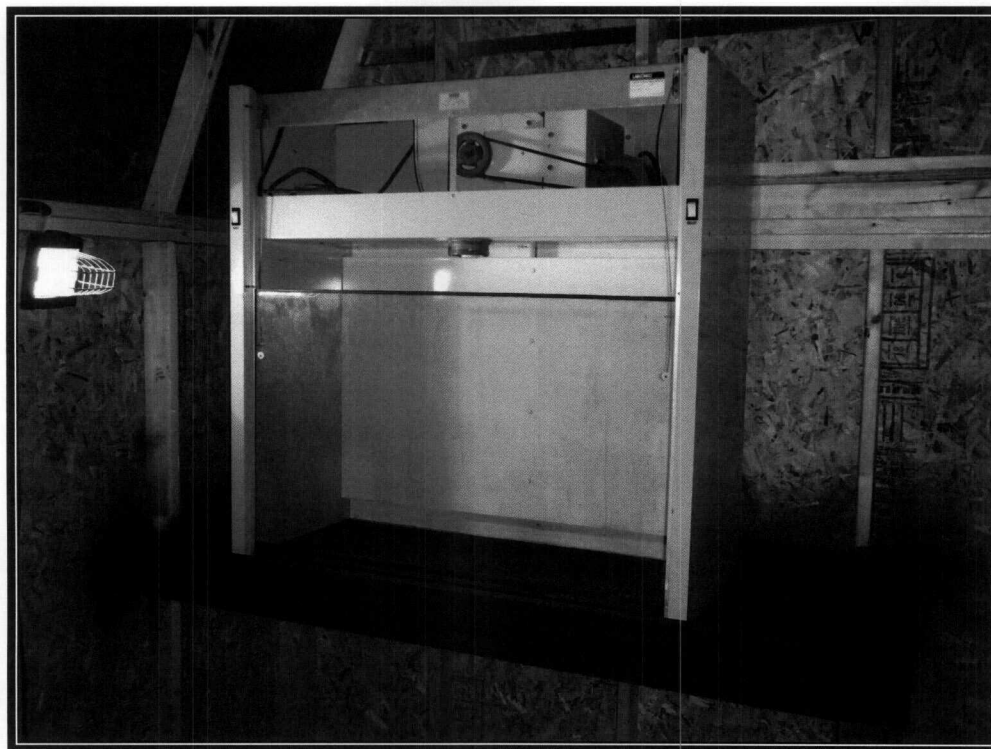
Photo 11: View of Vent Hood being installed for Mercury Filtering
