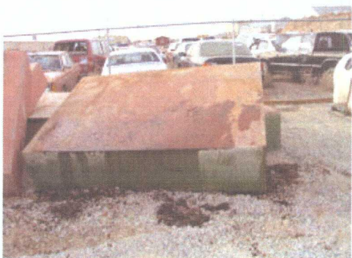
Photo 8: Discharge on to ground from containments.
