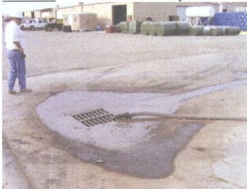
Photo 14: Sump in secondary containment area.
