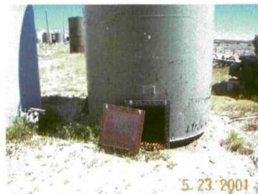
Tank bottoms spilling from manway of crude storage tank
