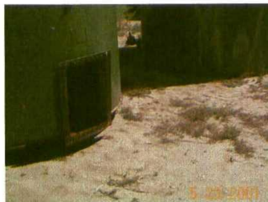
Crude oil storage tank from which sample was taken – note that no leaking has occurred.
