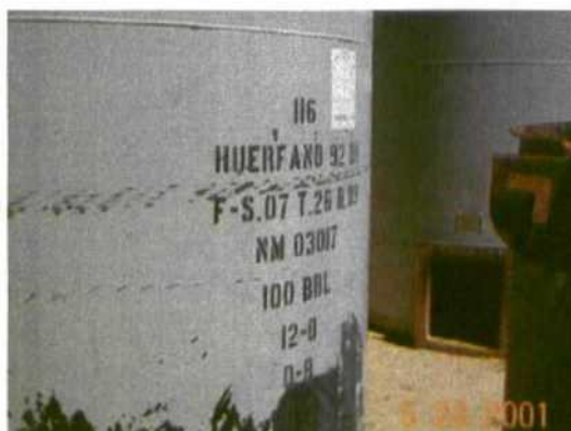
Owner labeled crude oil storage tank with location and well name.
