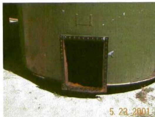
Open manway on crude oil storage tank Sample of tank bottoms taken from inside tank.
