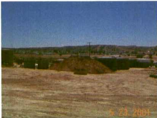
Cleaned area where previous staining was found. Contaminated soil pile to be removed for proper disposal.
