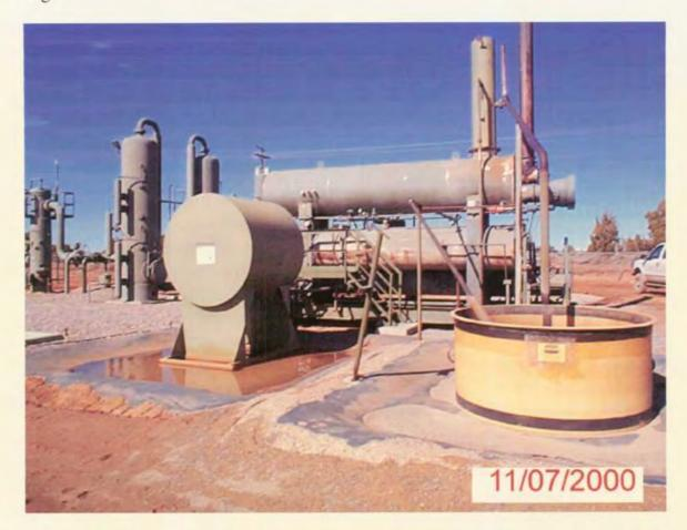
Picture #2- TEG Storage tank and De-hydrator waste water tank. Secondary liner is torn on both.
