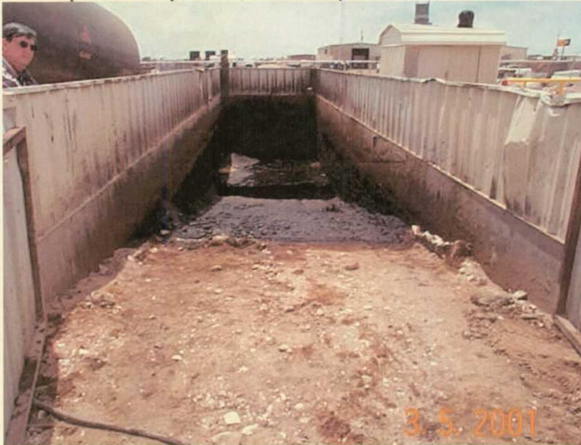
Pic # 2- Wash Out Pit constructed of concrete has no secondary liner.
