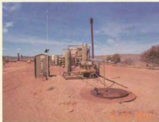
Pic #2 de-hydrator double wall sump
