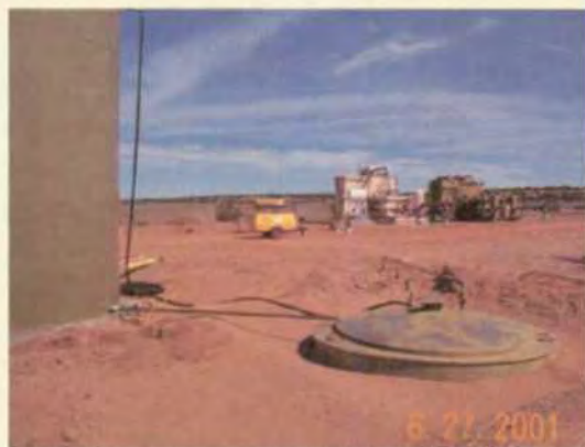
Pic #3 Waste water tank with double wall sump.
