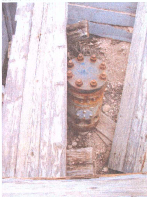
Photo 2: Bolted flange on protruding metal casing being surrounded by broken wooden box.
