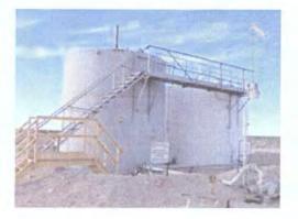
2) The sour tank is in service and similar to the above tanks, the secondary containment area is not lined. A 60-mil HDPE liner similar to No. 1 above is required to be installed within 90 days of this correspondence and the bermed area shall be constructed to contain at least 1.333... of the volume of the tank within the bermed area.
