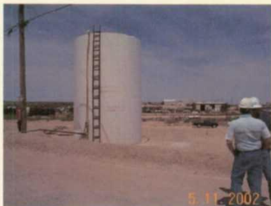
Picture #3- Fuel tank area-needs proper containment.
