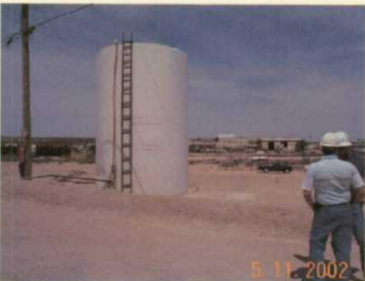
Picture #3- Fuel tank area-needs proper containment.
