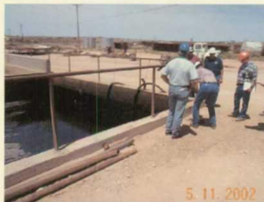
Picture #5- Frac tank wash-out pit. Inspecting leak detector.
