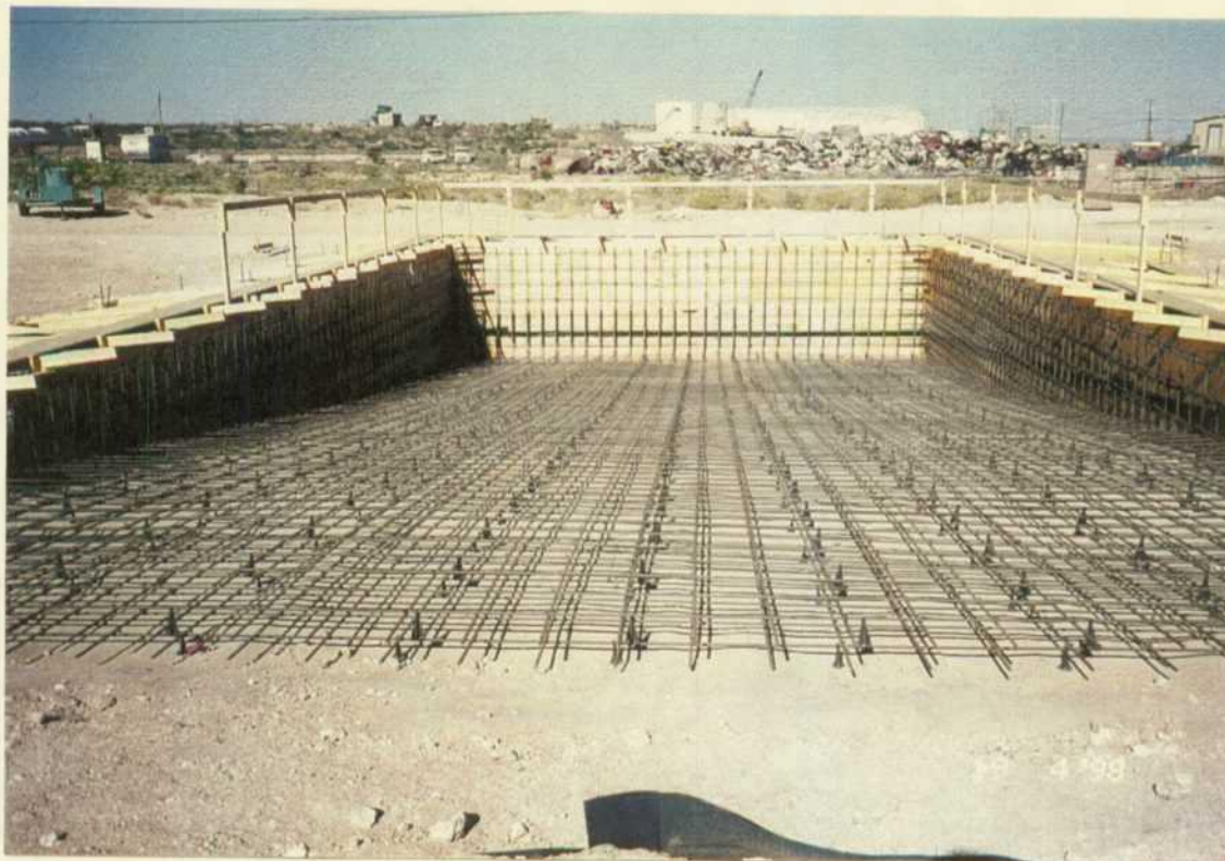
Photo Number: 5 Photographer: N. Jones Location: Rowland Trucking Company Subject: Close-up of rinsate pit under construction City/County: Carlsbad State: NM Date: 04/20/98 Time: 4:58 PM Weather: Sunny
