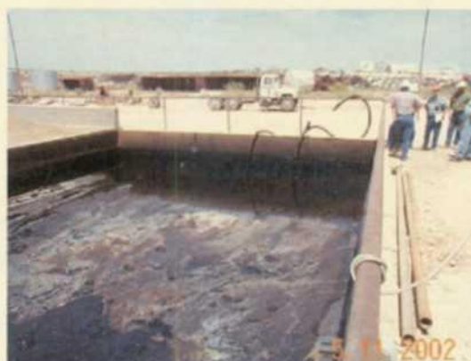
Picture #6 - Concrete wash-out pit with secondary containment and leak detection.
