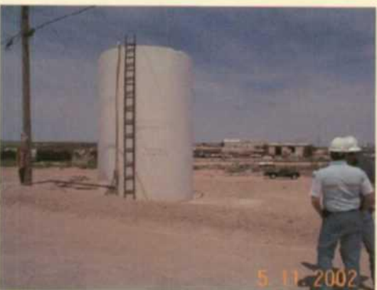
Picture #3- Fuel tank area-needs proper containment.
