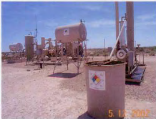
Picture #2- TEG & Glycol wastewater tank-both need containment.
