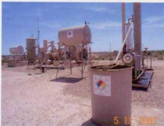
Picture #2- TEG & Glycol wastewater tank-both need containment.
