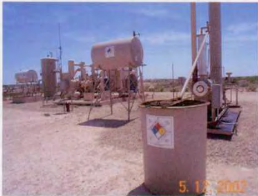
Picture #2- TEG & Glycol wastewater tank-both need containment.
