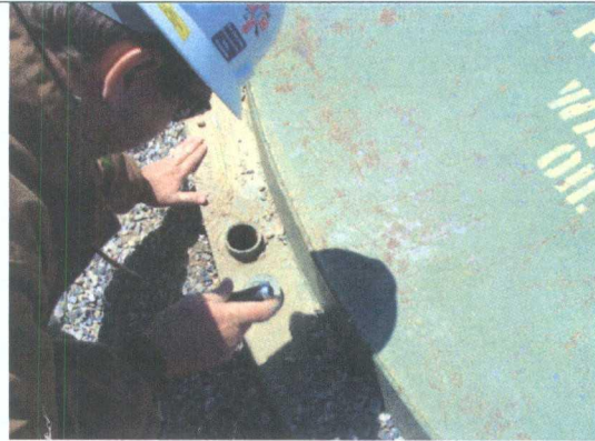
Photo 4: BGT (T509) verified WET leak detection system.
