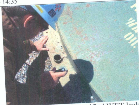
Photo 4: BGT (T509) verified WET leak detection system.
