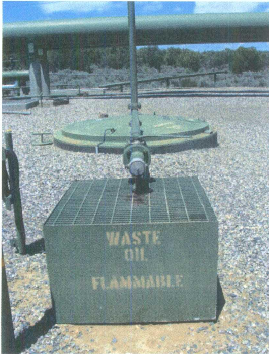
Photo 7: Catch bin for drain off of BGT.
