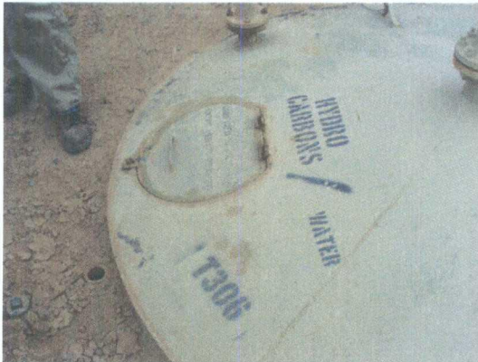
Photo 2: BGT (T306), for pigging fluids. Leak detection verified, WET.
