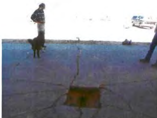
Wash bay with sump and drain going out to underground tank. Located on east side of shop building. Tank has no secondary containment. Owner indicated they are going to replace tank with one that has secondary containment.
