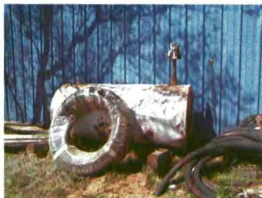
Southside of shop area Waste Oil Tank with no containment.
