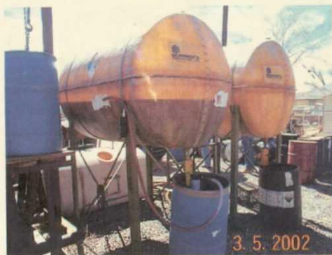
Tank area – Chaco Chemical – Farmington Unknown chemicals. No Containment.
