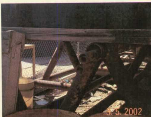
Different view under elevated drum storage deck. Note that plastic liner does not extend completely to limits of deck area.
