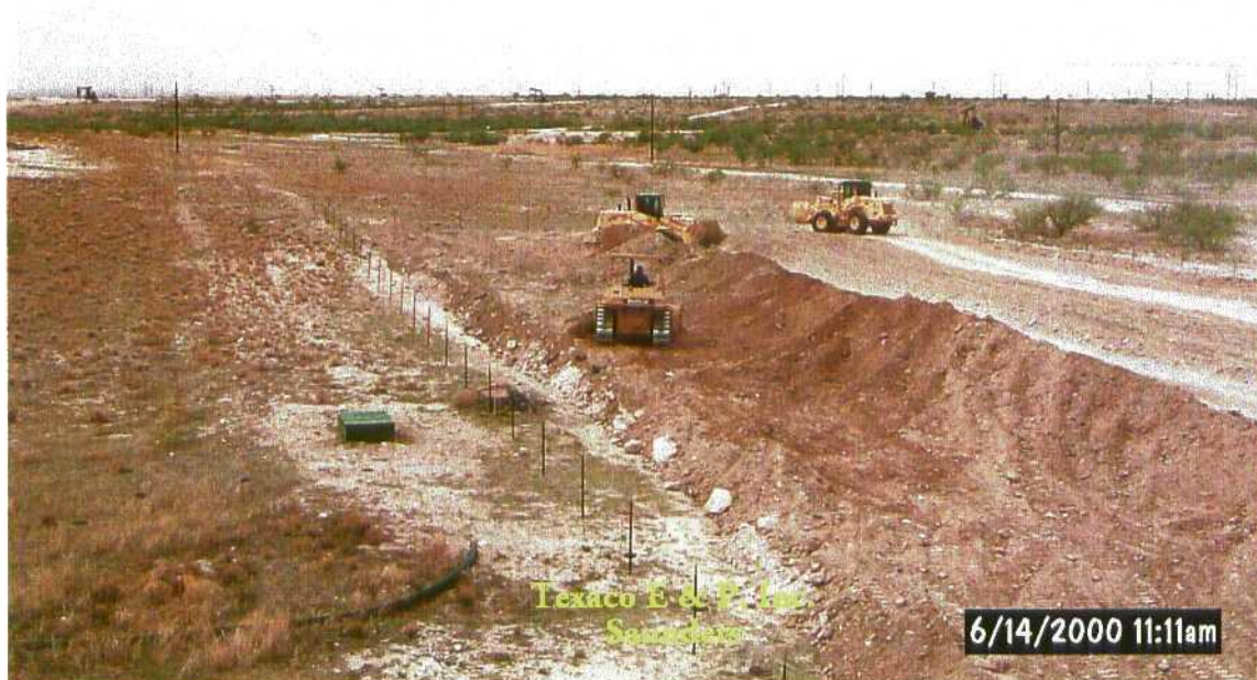
Moving tested and treated soil from Blending and Treating Area to Excavation
