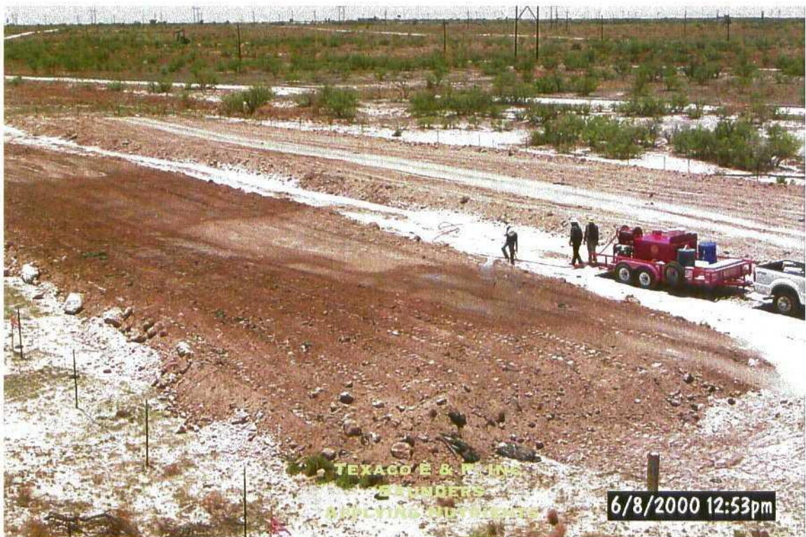
Nutrients being applied to blended and tested lift
