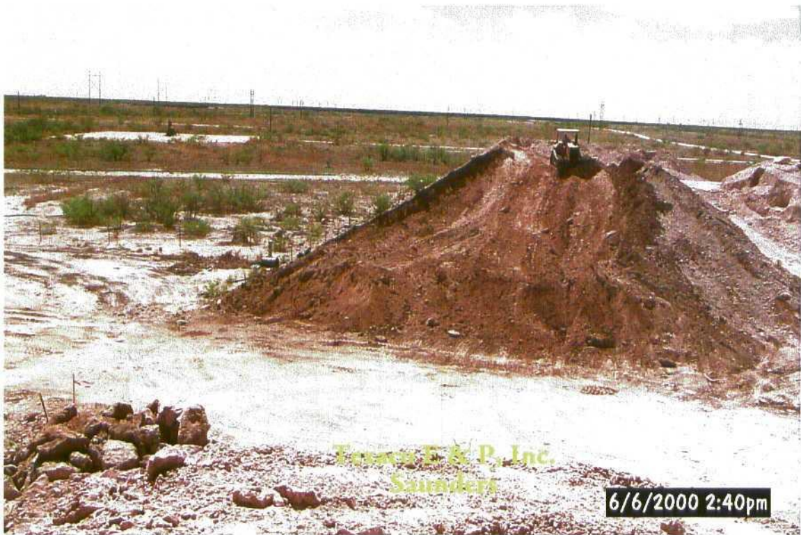
Pushing soil to the loaders
