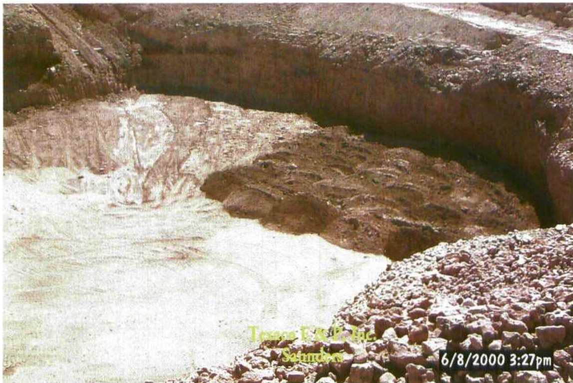
Treated soil emplaced in excavation bottom
