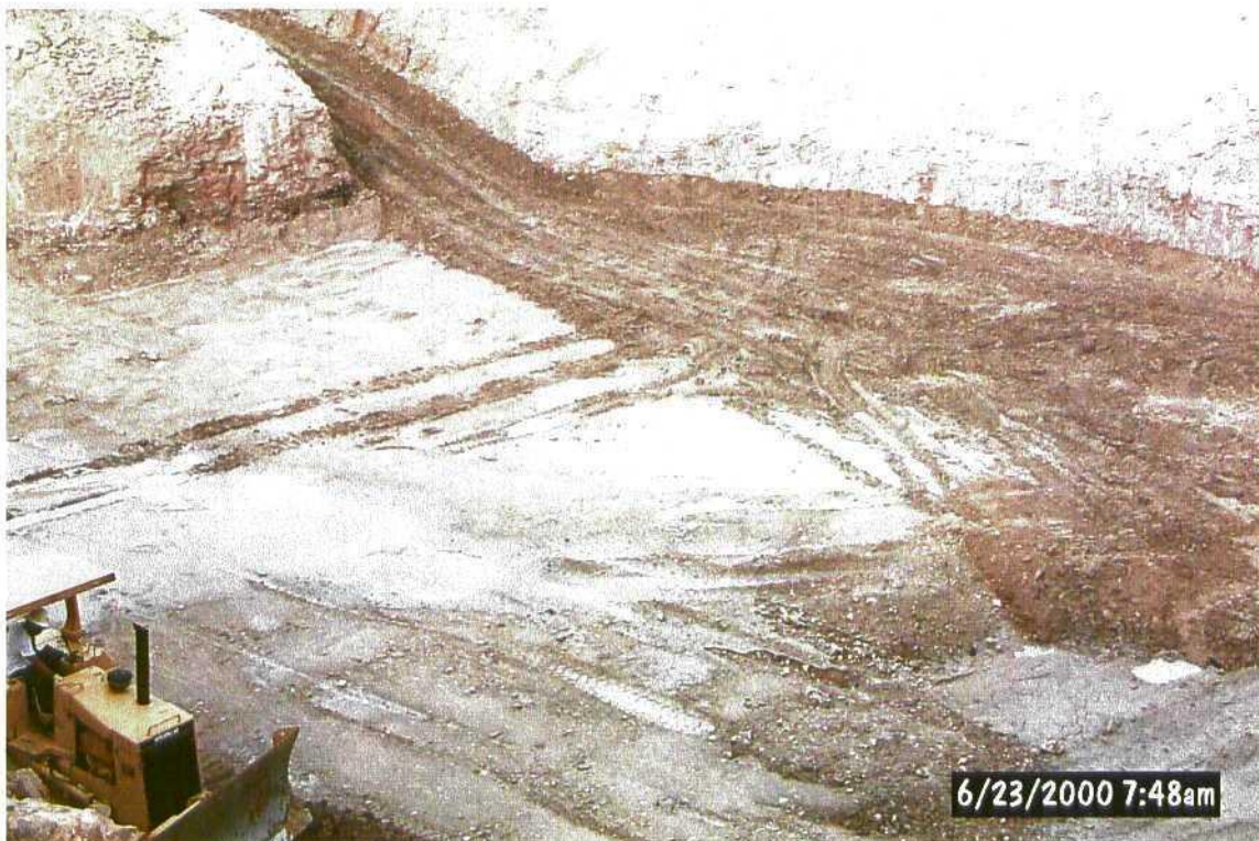
Spreading backfill (liquid is rain water)
