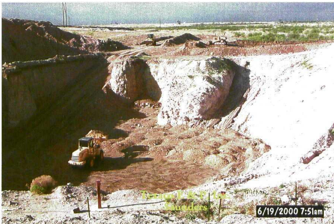
Emplacing tested soil from the Blending/Treating Area.
