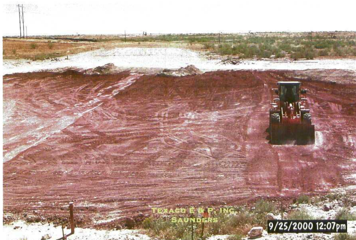
Clay barrier installation and compaction
