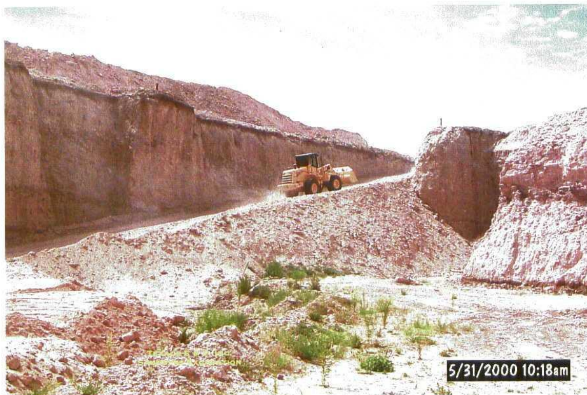
Backfilling initial 2' Lift
