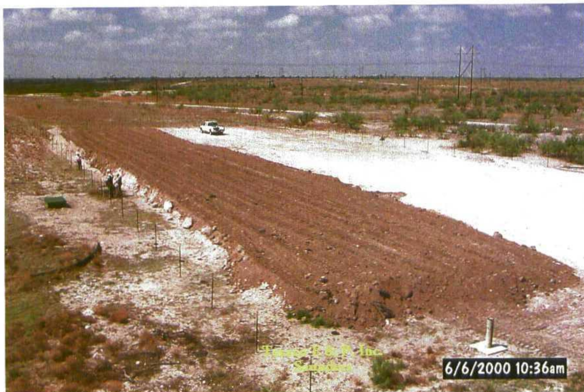
Blending and Treating Area – Lift ready for sampling
