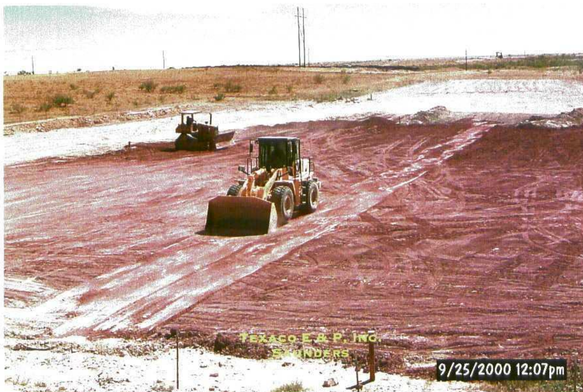
Clay barrier installation and compaction
