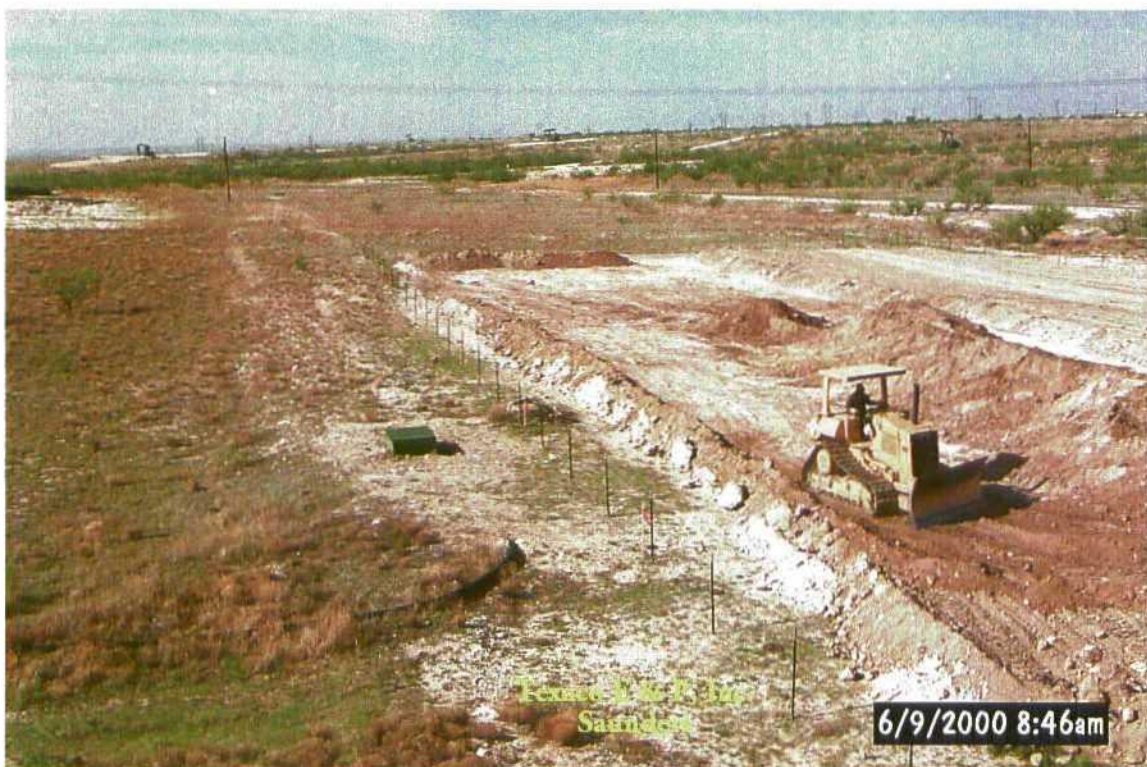
Treated soil being pushed for loading and emplacement
