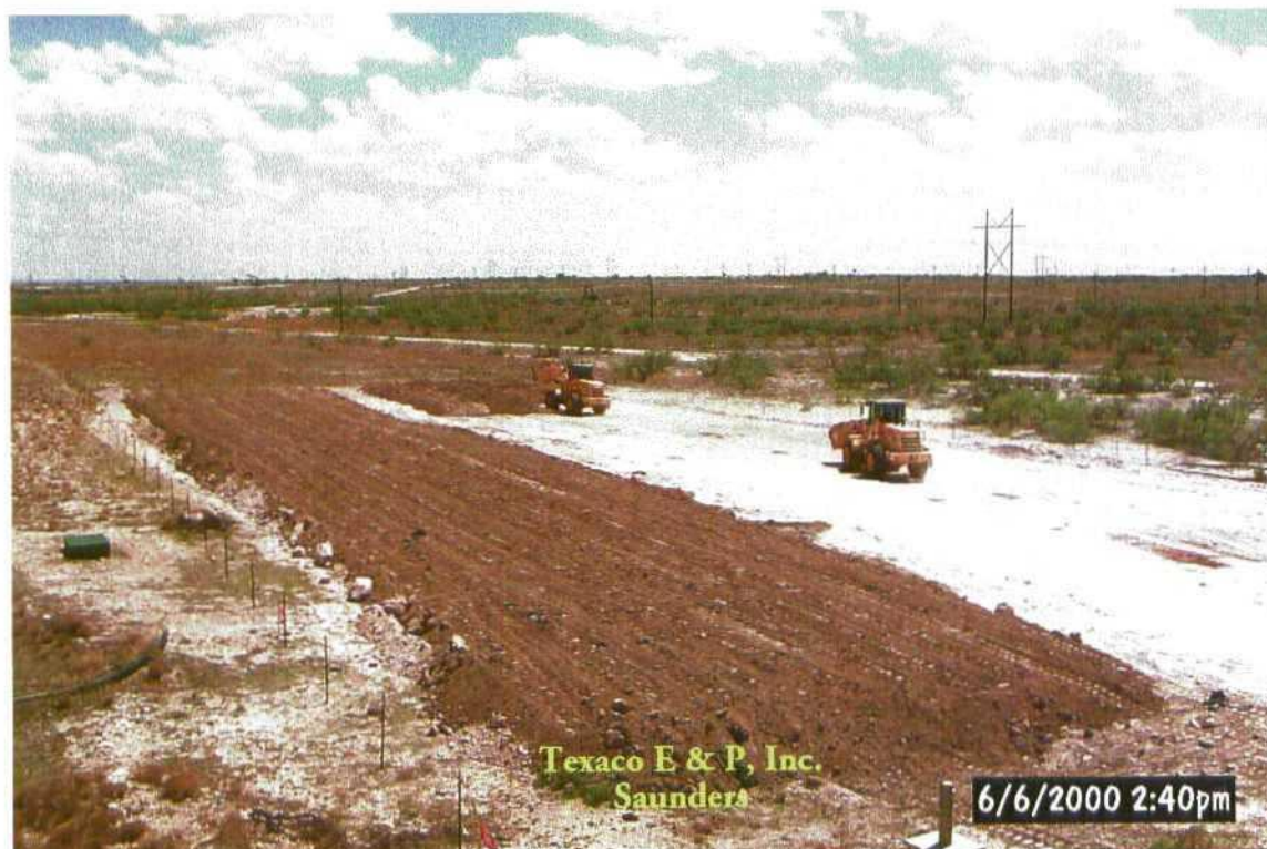
Contaminated soil being moved into Blending and Treating area. Two soil lifts, i.e., East and West, compensated for lag time between sampling, receiving results, treating, and backfilling.
