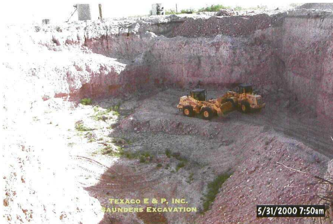
Backfilling initial 2' Lift
