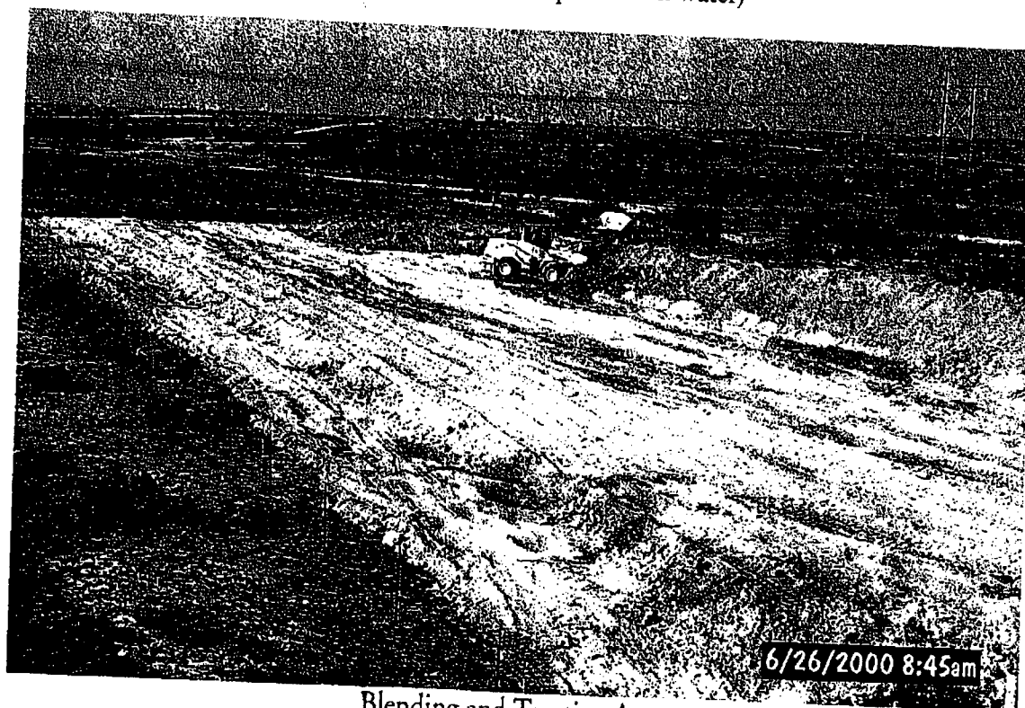
Spreading backfill (liquid is rain water)
