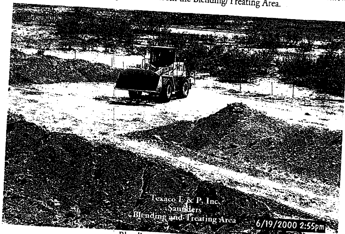
Emplacing tested soil from the Blending/Treating Area.
