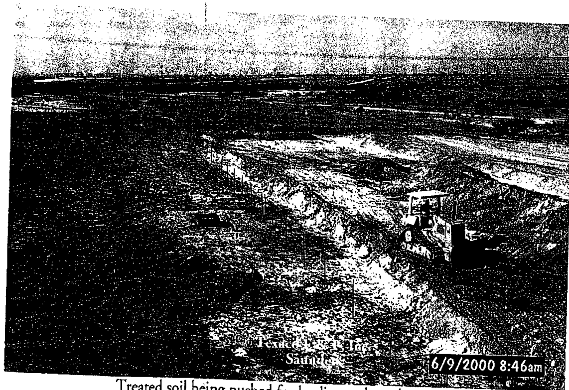
Treated soil emplaced in excavation bottom
