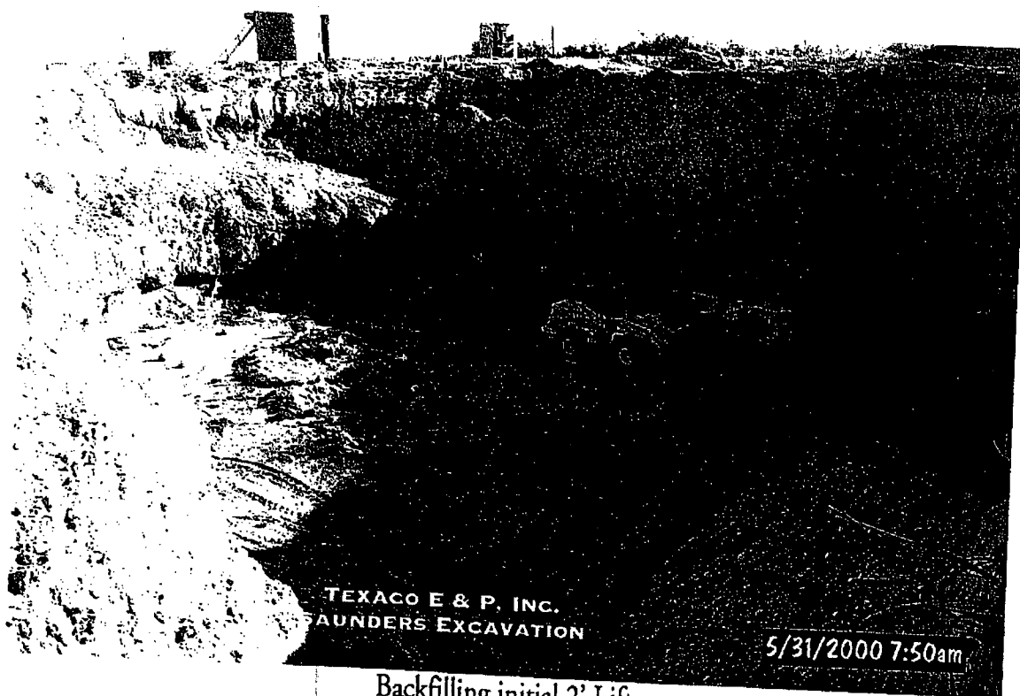
Backfilling initial 2' Lift
