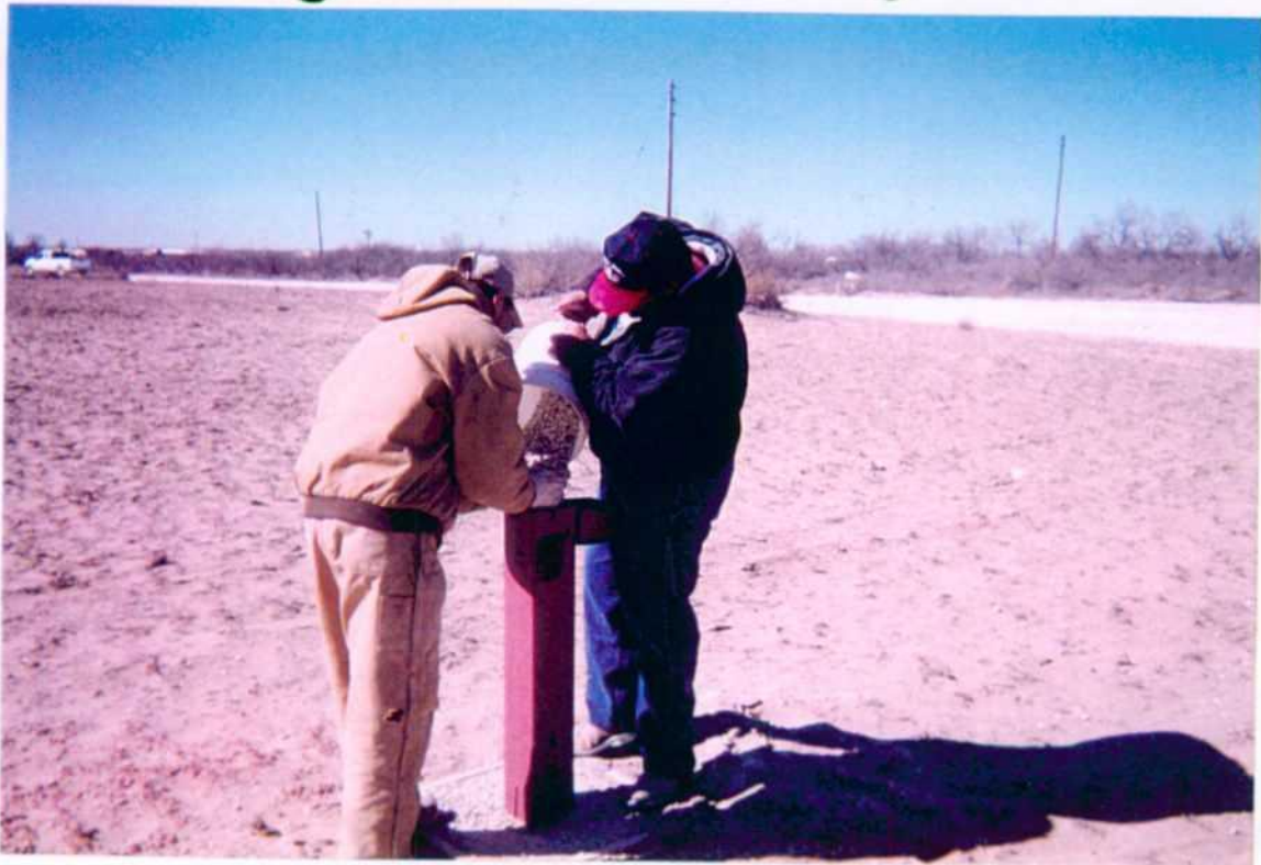
Photo 3: Grouting of monitor well MW-2.
