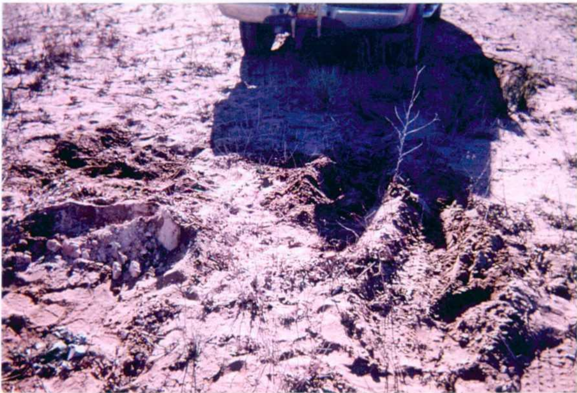
Photo 8: Completed removal of monitor well MW-3.
