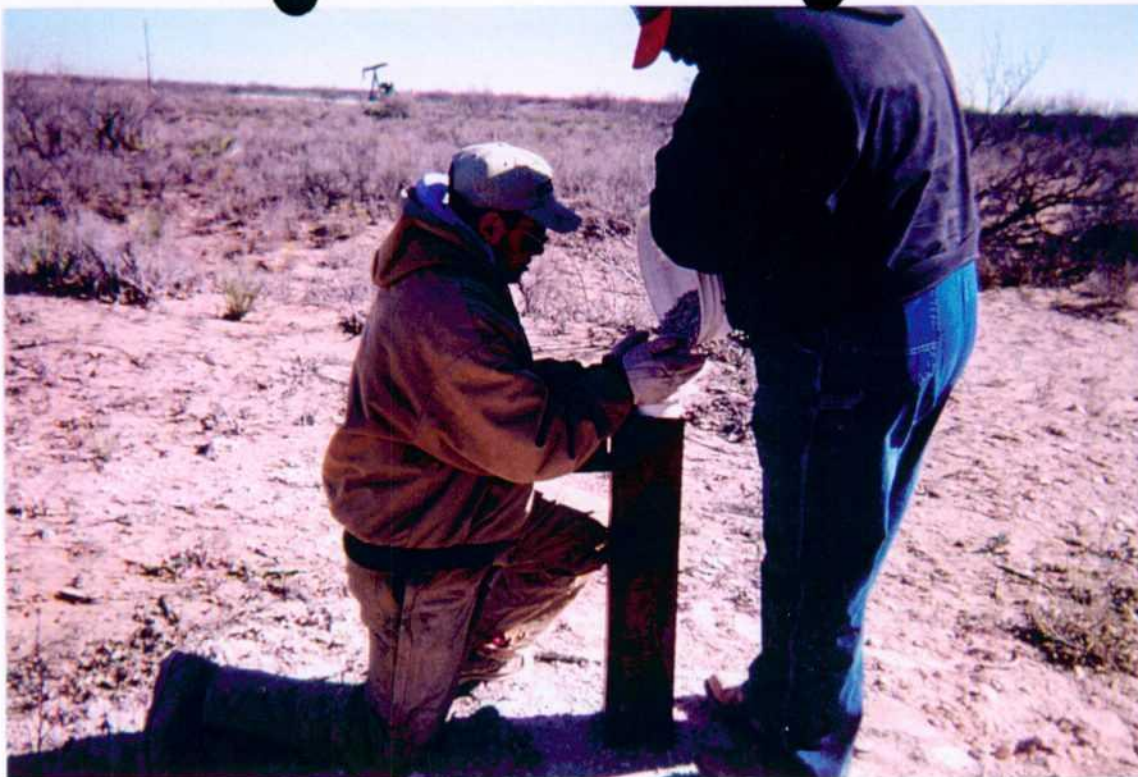
Photo 5: Grouting of monitor well MW-3.
