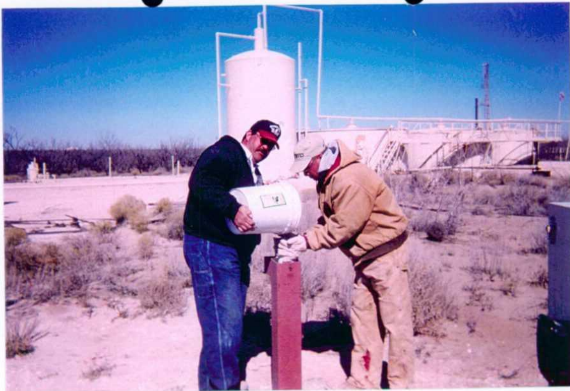
Photo 1: Grouting of monitor well MW-1.
