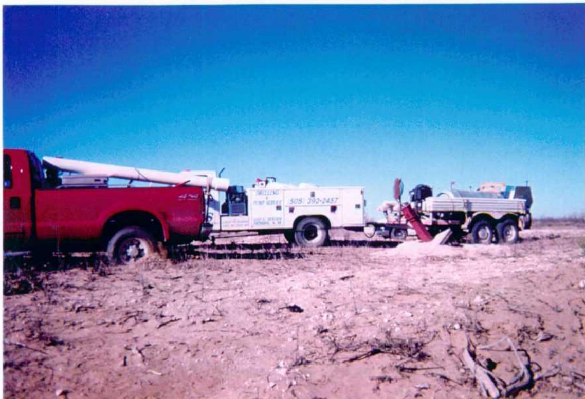
Photo 6: Removal of monitor well MW-3
