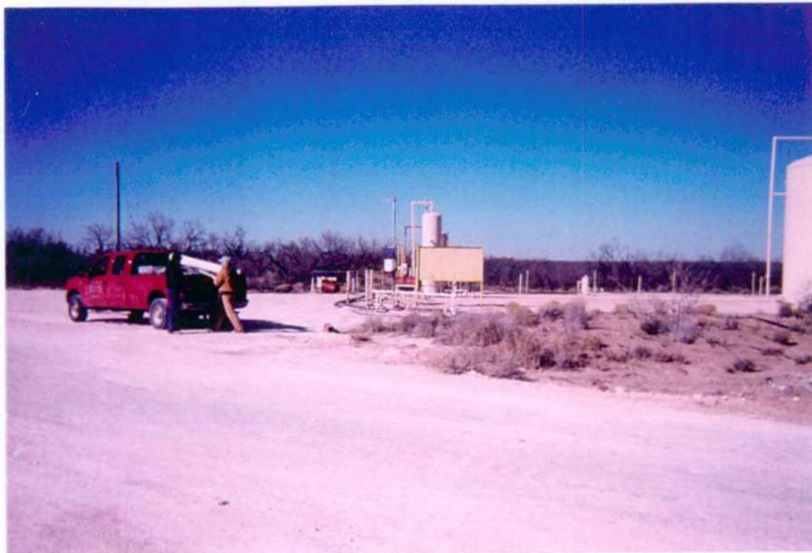
Photo 2 : Removal of monitor well MW-1.
