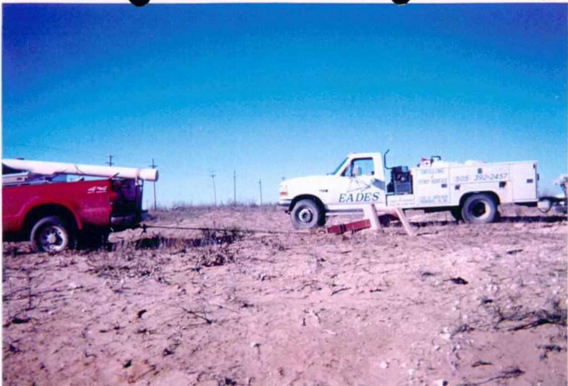
Photo 7: Removal of monitor well MW-3.
