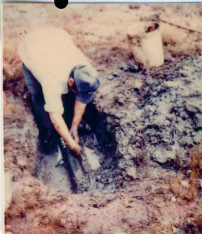
Fig. 2 Patching a leak. Dirt removed from around the pipe is saturated with brine and oil.
