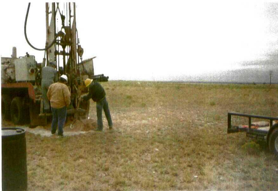
View facing south showing drilling operations at MW-3 (left foreground) located approximately 650 feet upgradient of the former SWD pit (right background).
