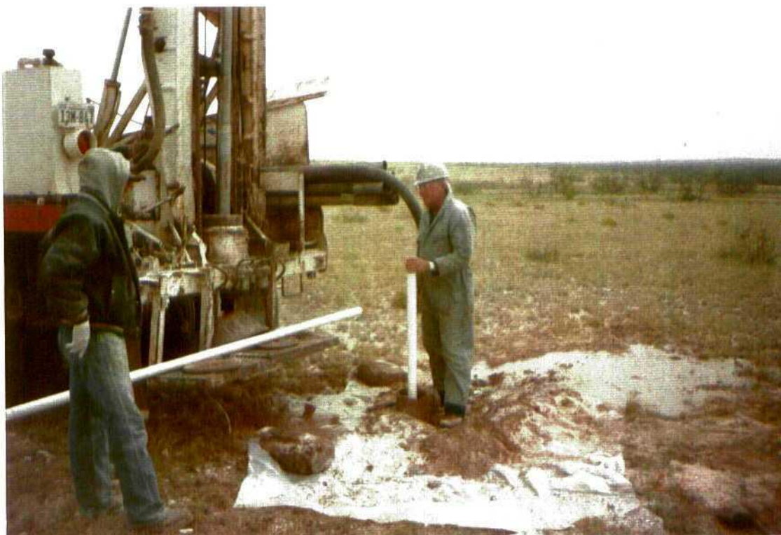
View showing monitoring well installation for MW-4 (facing southeast). MW-4 is located approximately 850 feet downgradient (southeast) of the former SWD pit.
