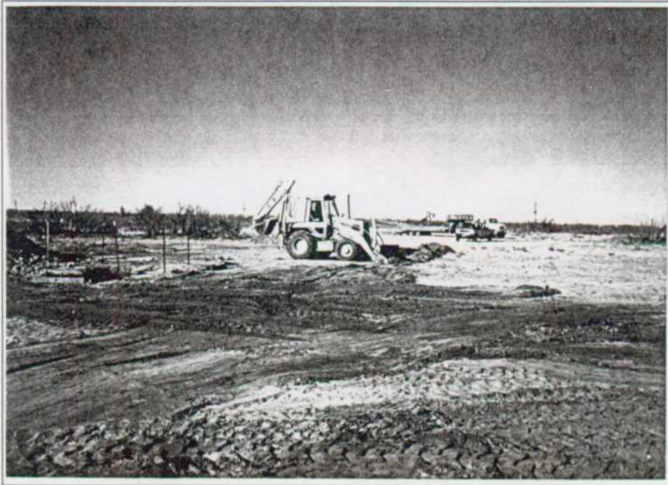
Backfilling of trenches.
