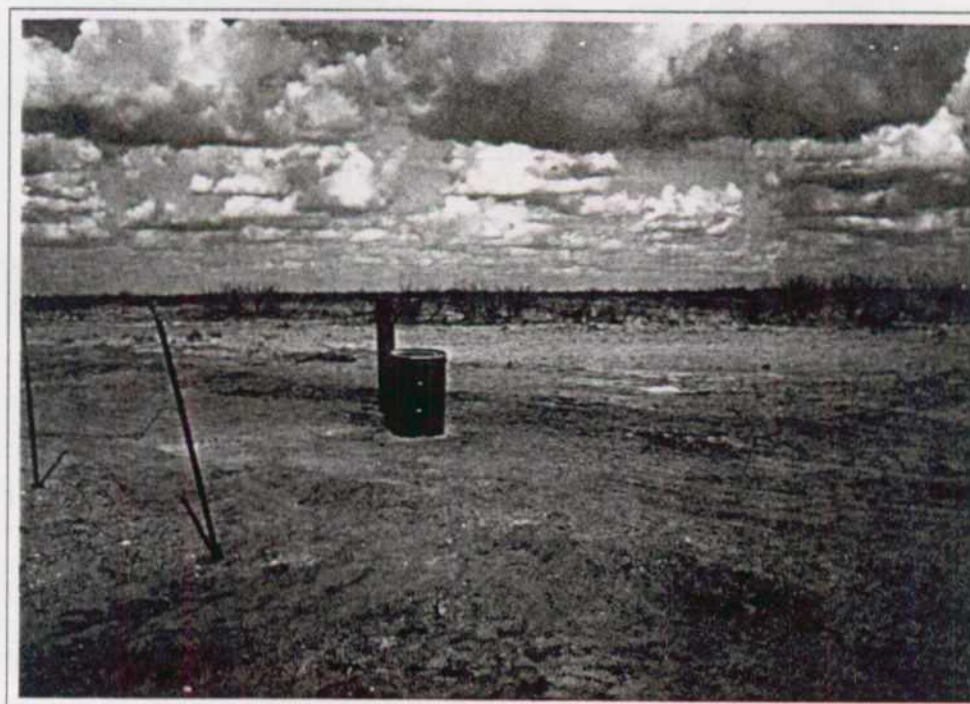
Completed MW-1 with sample drum.
