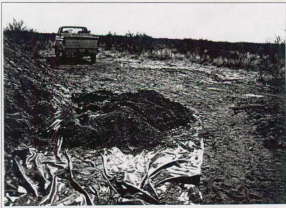
Drill cuttings stockpiled on plastic.
