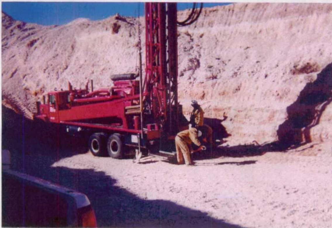
Photo 1: Drilling of Temporary Monitor Well TMW-1.
