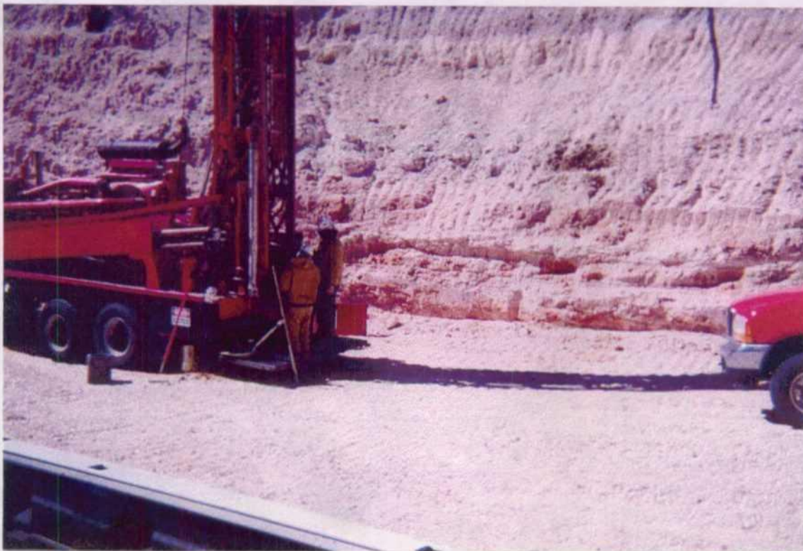
Photo 3: Drilling of Temporary Monitor Well TMW-1.
