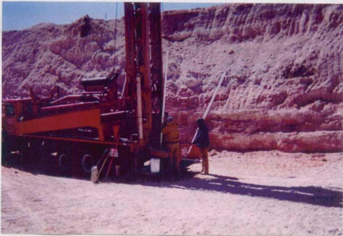
Photo 5: Installation of piping for Temporary Monitor Well TMW-1.
