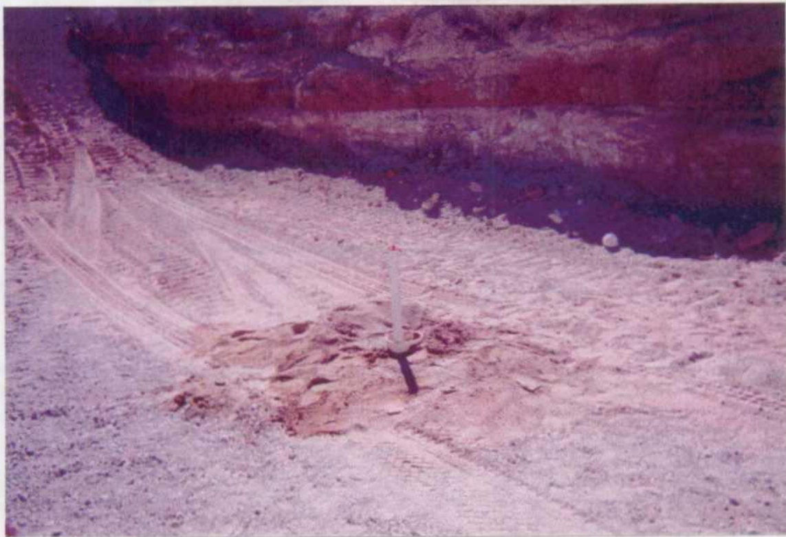
Photo 6: Completed Temporary Monitor Well TMW-1.
