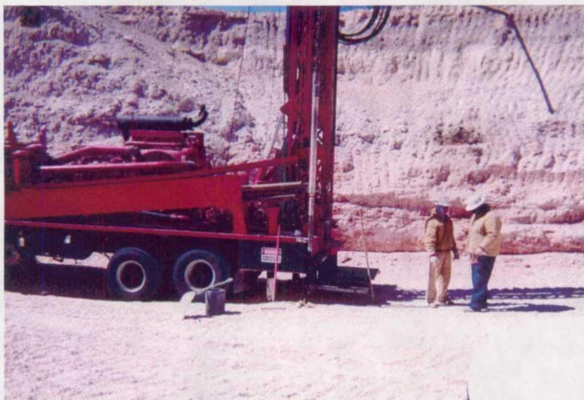
Photo 2: Drilling of Temporary Monitor Well TMW-1.
