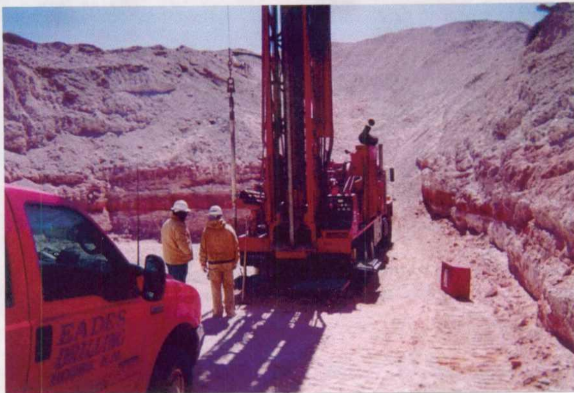
Photo 4: Drilling of Temporary Monitor Well TMW-1.
